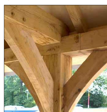
OAK FRAME DETAILING. KILN DRIED GREEN OAK DETAILS
