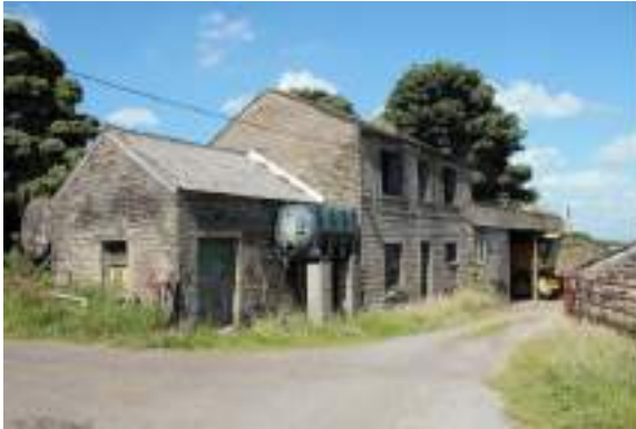
Figure 19: Former Yew Tree Farm farmhouse (derelict)
