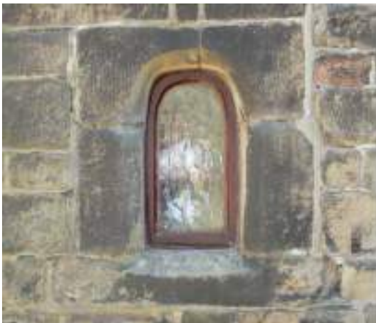
Figure 17: Small arched window on 55 The Village
