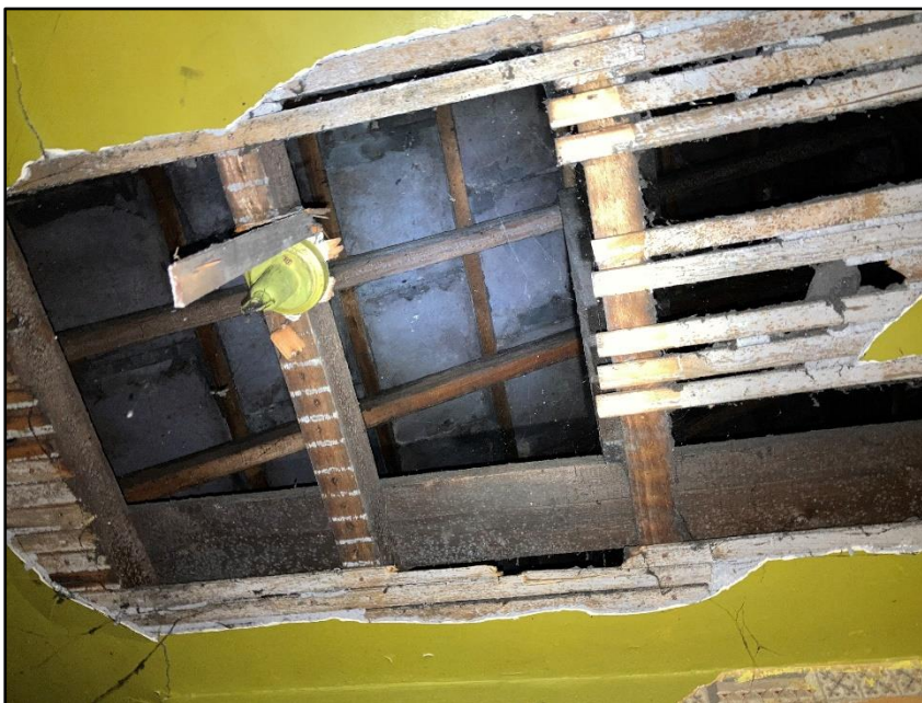
Photograph 27 showing the underside of one of the roof sections
