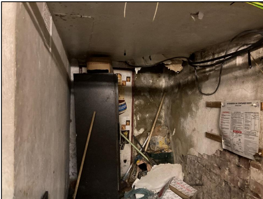
Photograph 21 showing the basement
