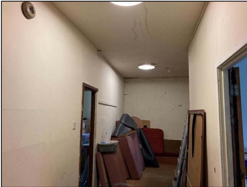
Photograph 22 showing the interior of the building
