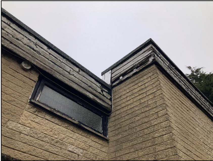
Photograph 20 showing a section of bargeboards
