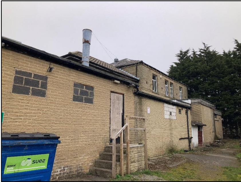
Photograph 14 showing the exposed masonry across the rear of the property
