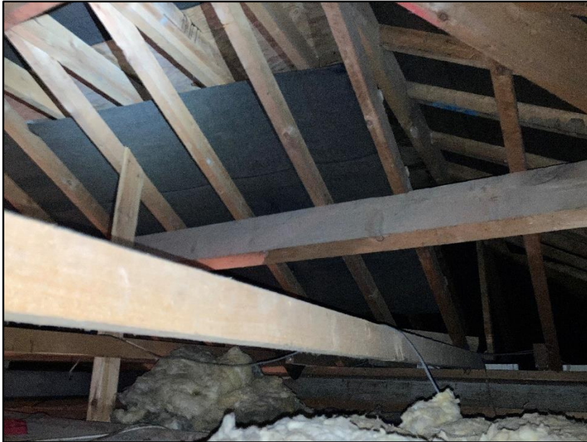
Photograph 26 showing one of the roof voids
