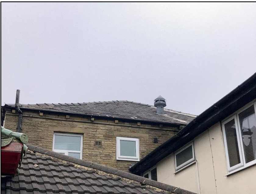
Photograph 17 showing a section of roof
