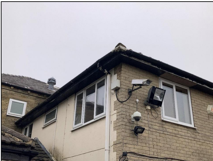
Photograph 15 showing the exterior of the building
