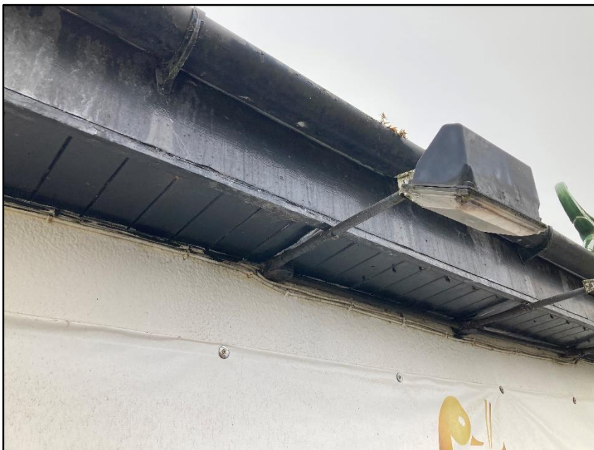
Photograph 19 showing a section of bargeboards and soffits
