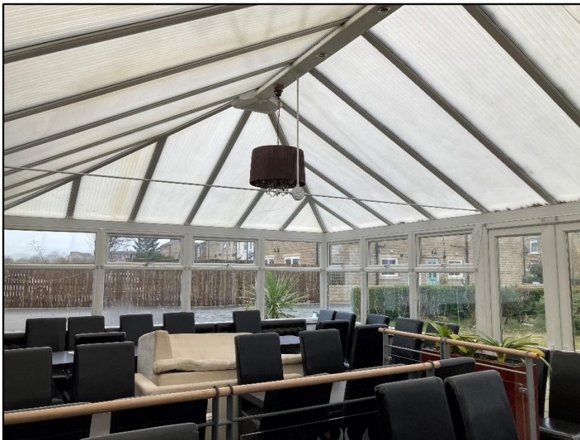
Photograph 23 showing the interior of the building
