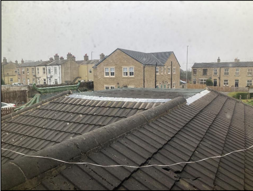
Photograph 16 showing a section of roof
