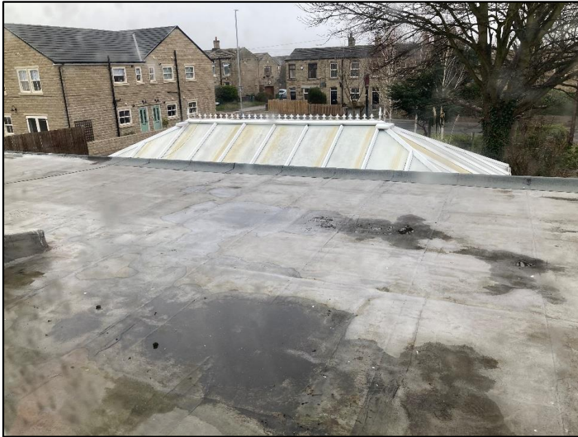
Photograph 18 showing a section of roof
