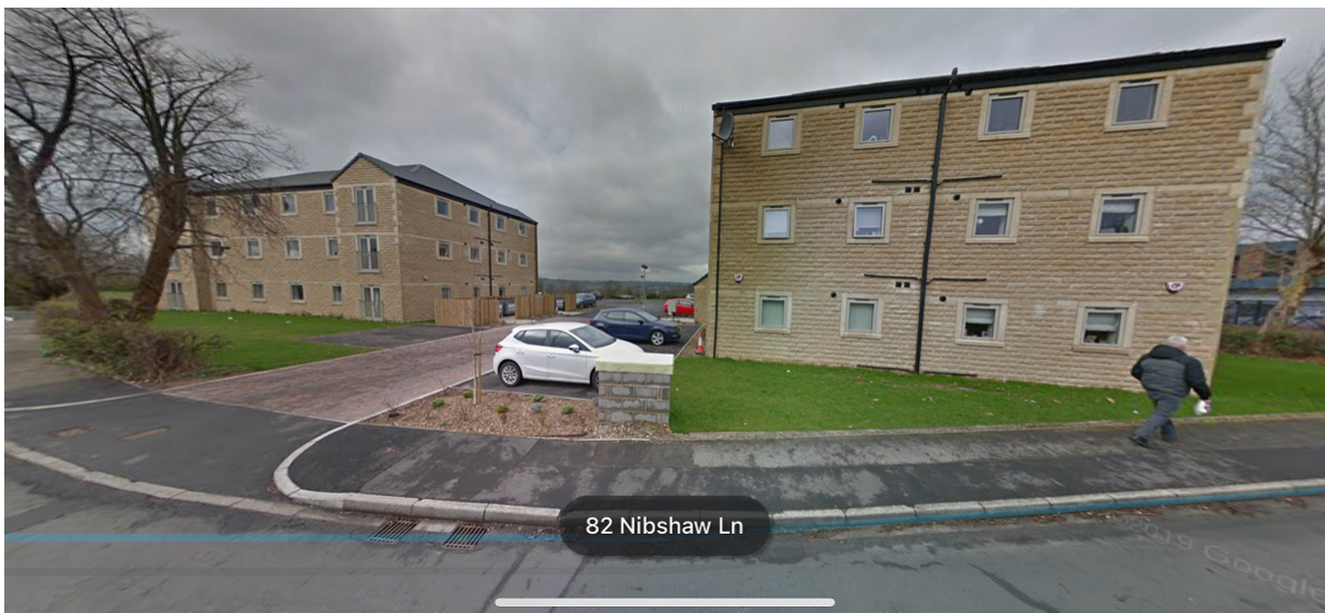
View of the side of the larger 24 apartment block and the rear of the smaller 12 apartment block
