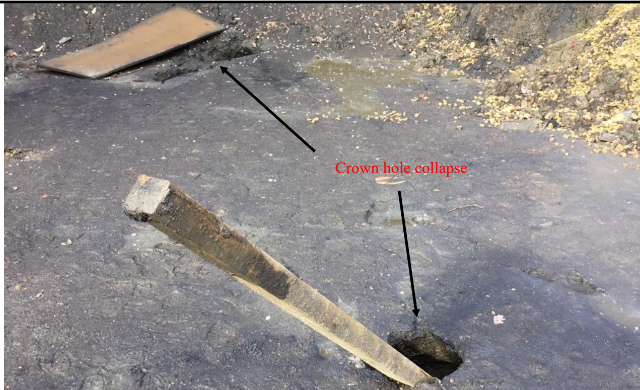
Photo 1: Upon arrival at site. Timber went approximately 2.5m to 3m into the hole before refusal.
