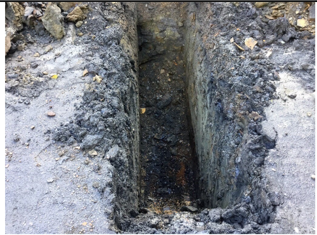
Photo 6: Intact coal at TP05.
