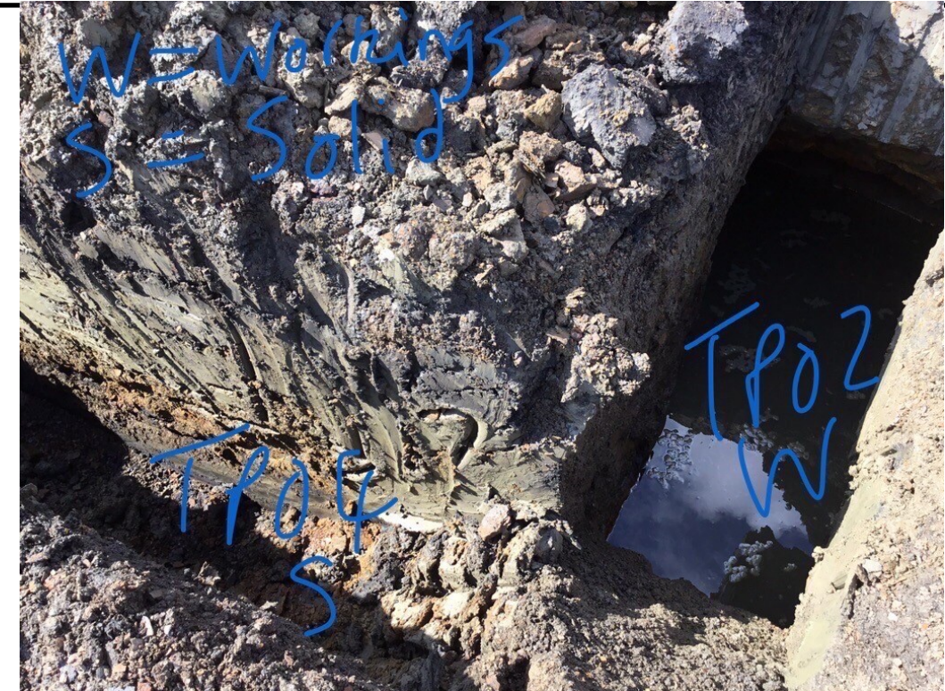
Photo 3: Example showing coal workings (flooded) at TP02 in comparison to solid ground at TP04.
