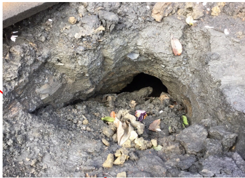
Photos showing ground conditions upon arrival at site. Roofs had begun to collapse.
