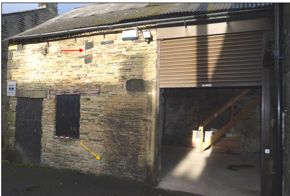
Photograph 15: Apertures to south elevation (facing north west) and construction breaks (indicated by red and yellow arrows). Scale 0.5m.
