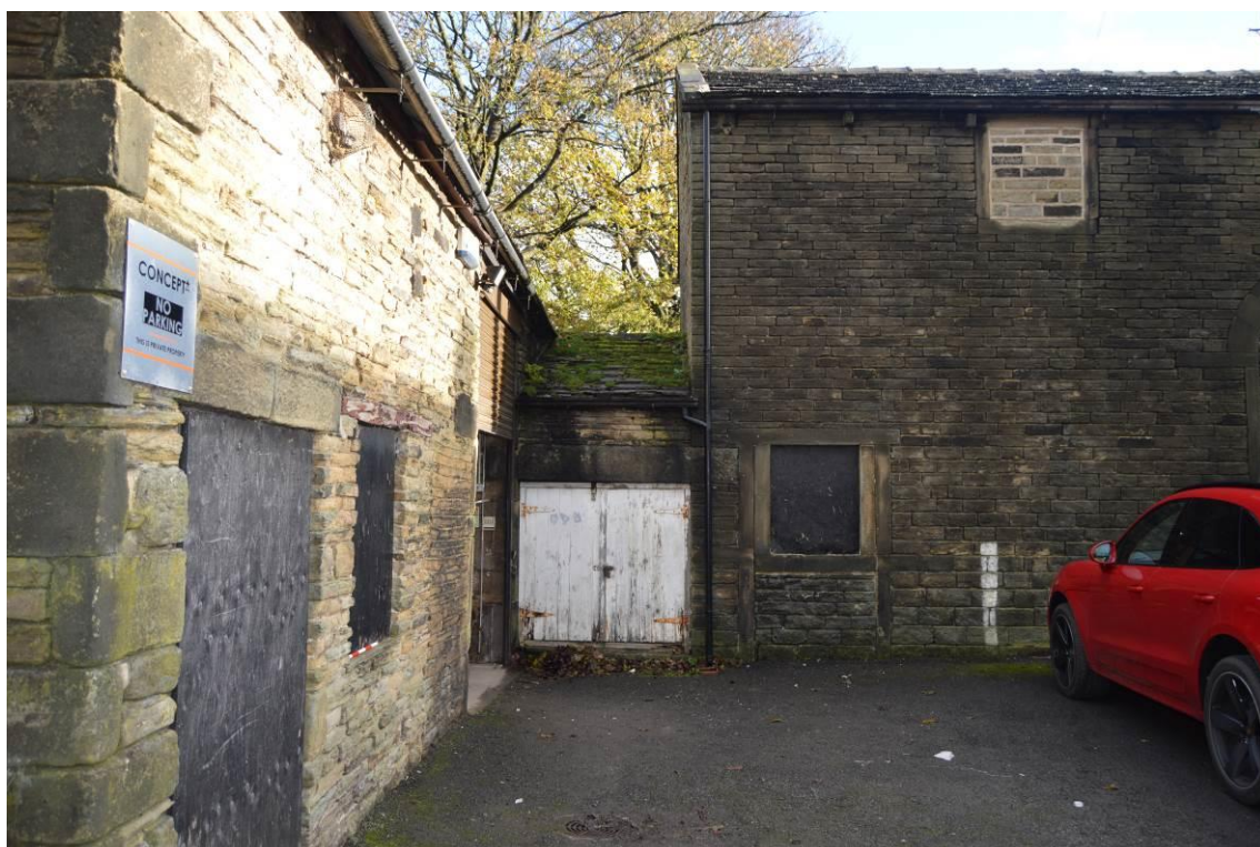
Photograph 24: Building 2 adjoining the two barns (facing east).
