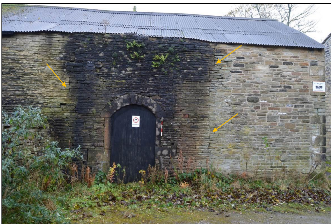
Photograph 14: North wall (facing south) with stone arched door and construction breaks (indicated by yellow arrows). Scale 0.5m.
