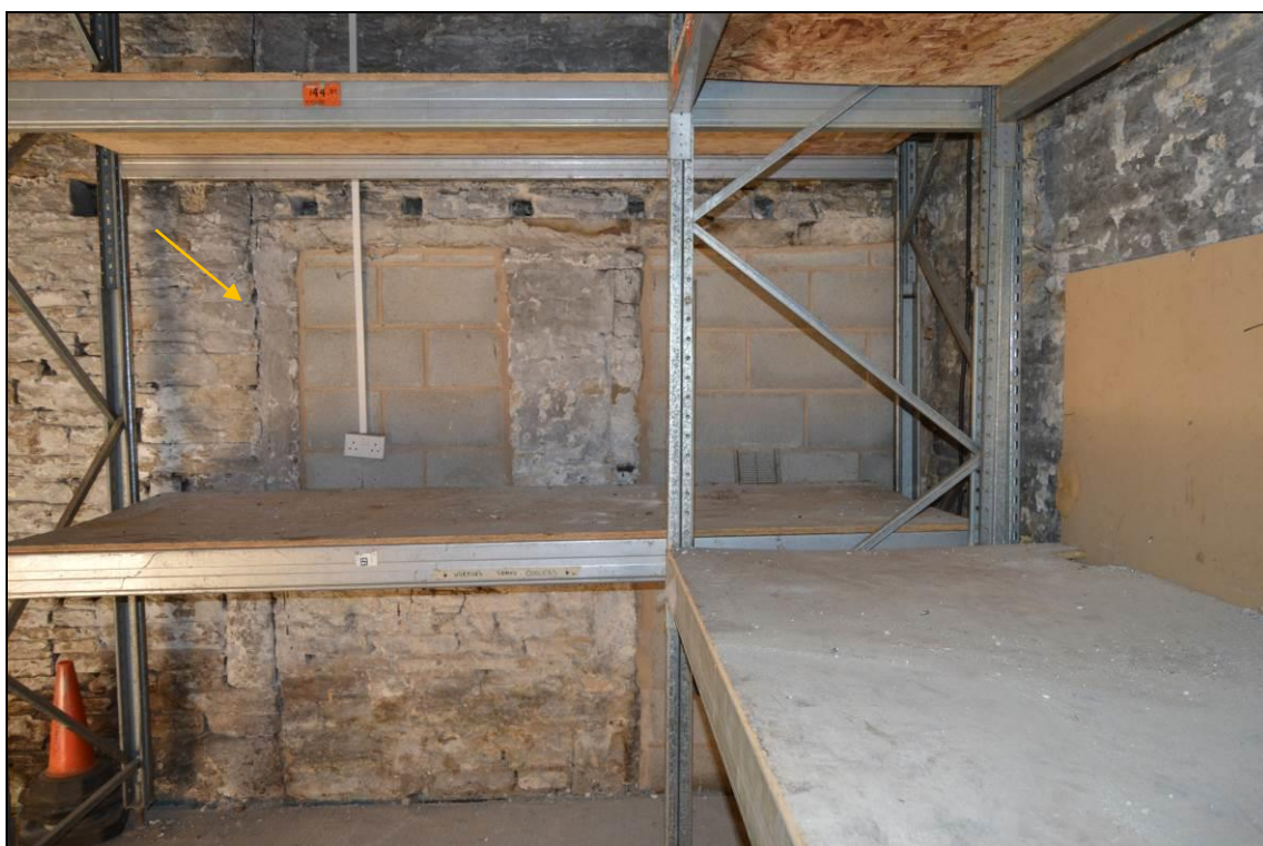
Photograph 16: Internal face of the barn's south elevation. Note construction break (indicated by yellow arrow) and joist slots.
