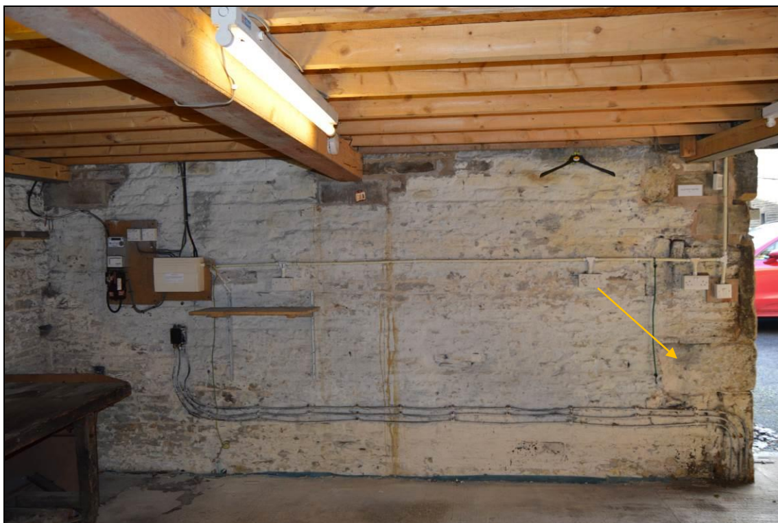
Photograph 17: Internal face of the barn's south elevation with quoin stone jamb indicated by yellow arrow: (facing south).
