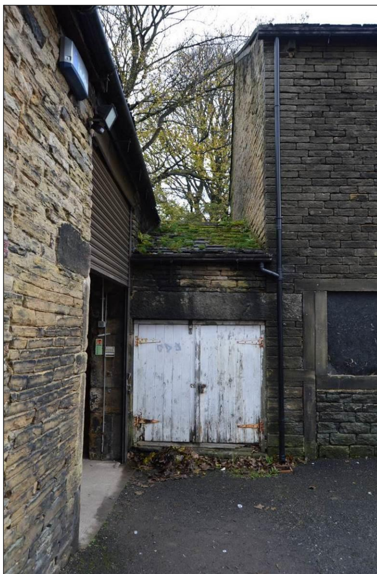
Photograph 23: Building 2 from the rear yard.
