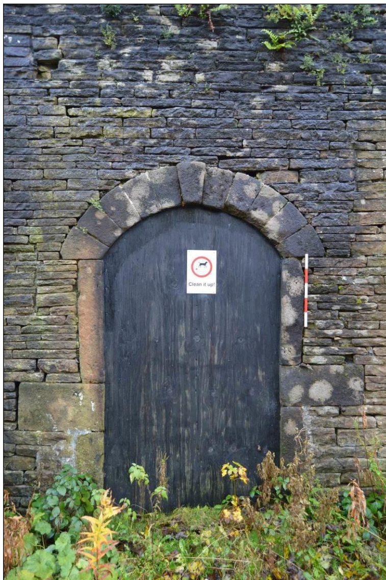
Photograph 12: North, field wall (facing south), with blocked stone framed doorway. Scale 0.5m.
