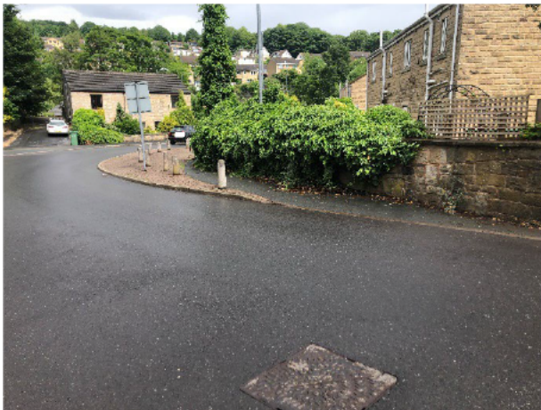
View at the bottom of Smithy Place where the footway begins – note the reduced visibility at the crossing point
