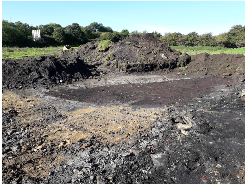
Figure 3.3.2; Mine Entry 417427-014, excavation area
