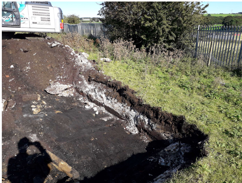
Figure 3.3.3; Lime material within excavation area
