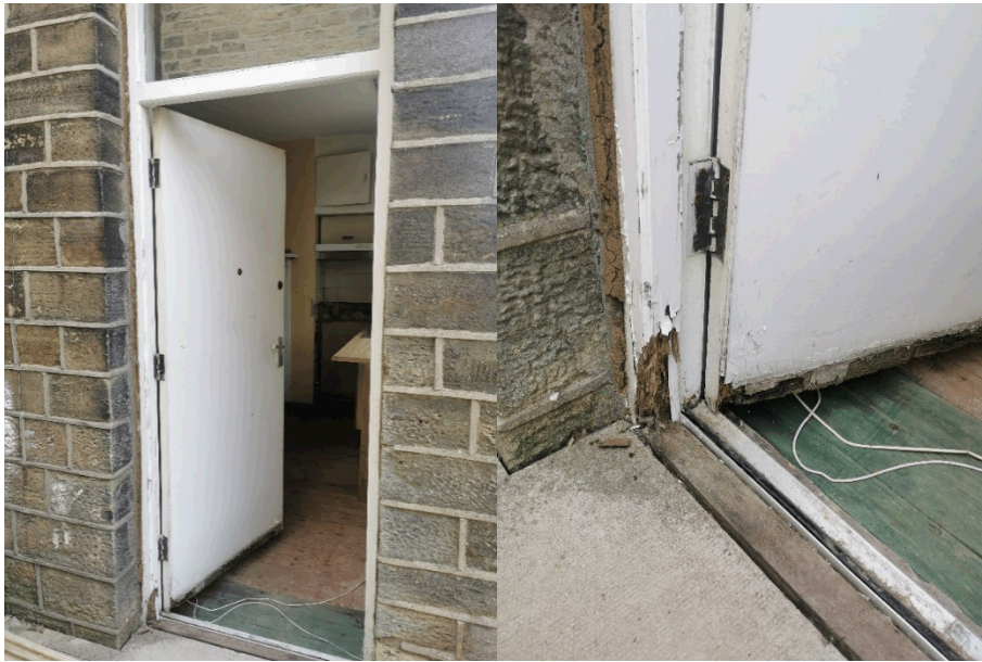
Photograph 6 – External rear door
