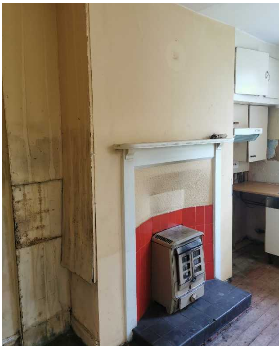
Photograph 5 - Kitchen Chimney stack
