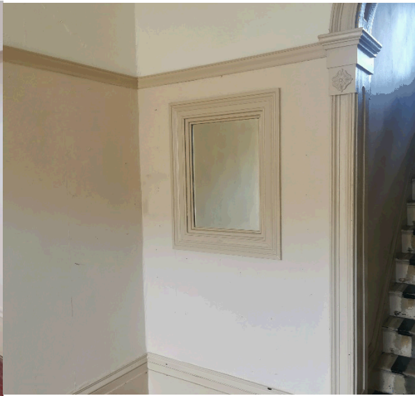
Photograph 4 - Proposed doorway location
