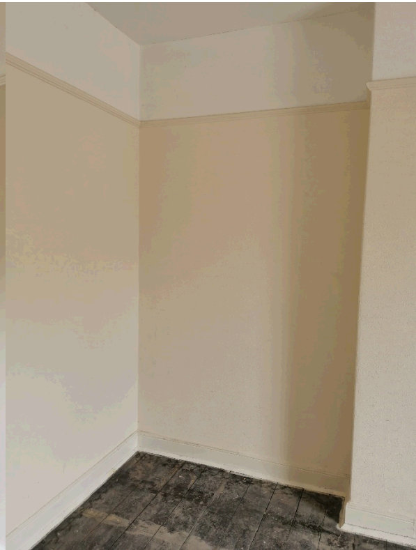
Photograph 13 - Bedroom 4 Ensuite location
