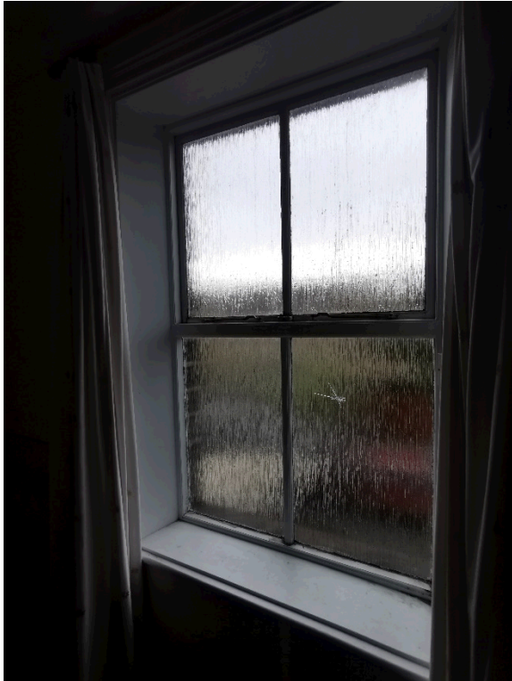
Photograph 15 – First Floor window
