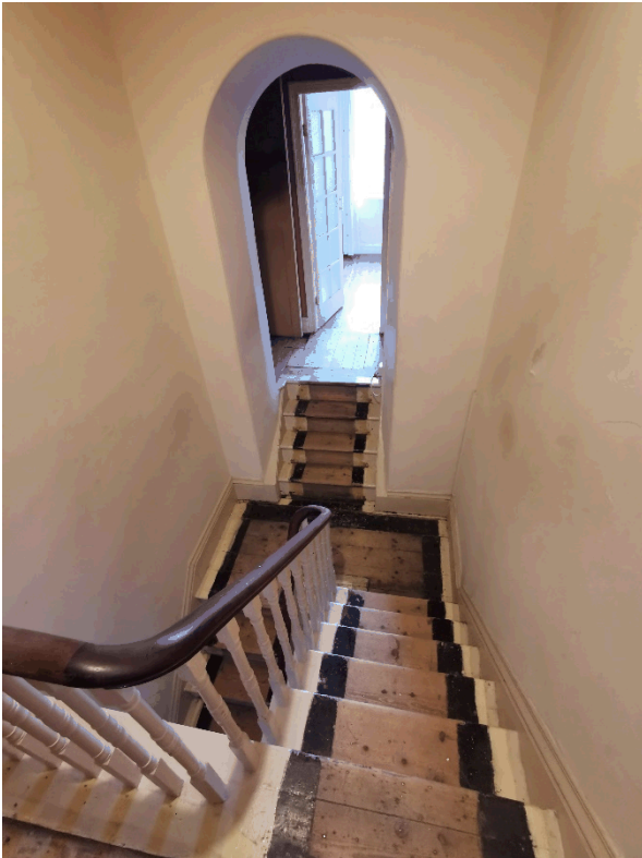
Photograph 8 - Staircase mid landing
