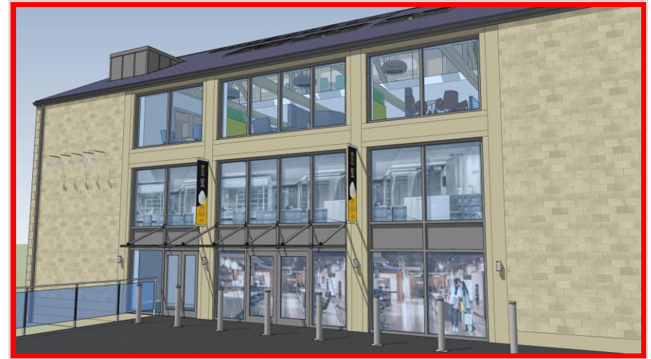
North facing elevation from St. John's Place
