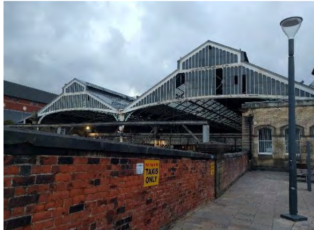
Figure 4-18 Preston (roofs constructed 1879-80)
