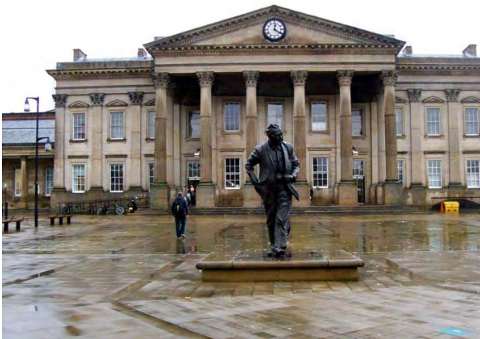
Figure 3-3 Front principal elevation of Station
