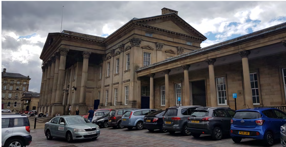
Figure 3-9/10/11/12 Main station building and warehouses
