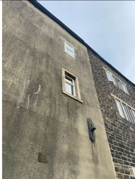
External side lounge window (Ground floor/first floor to back elevation) The window is the lower one
