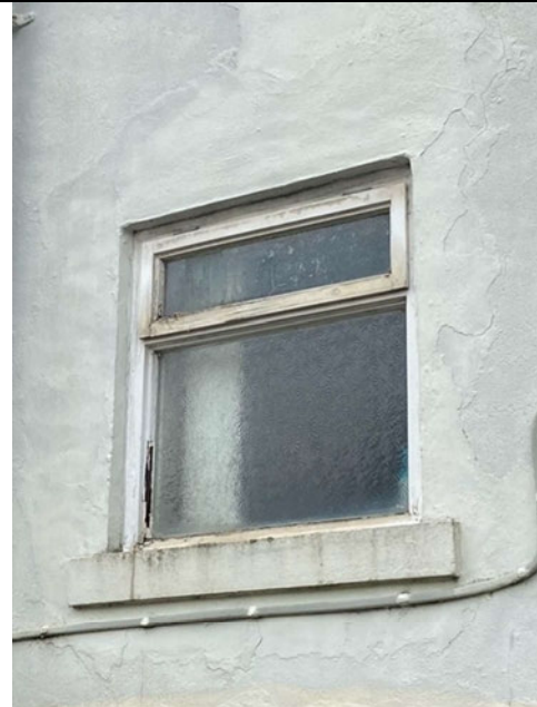
External Bathroom (street view)
