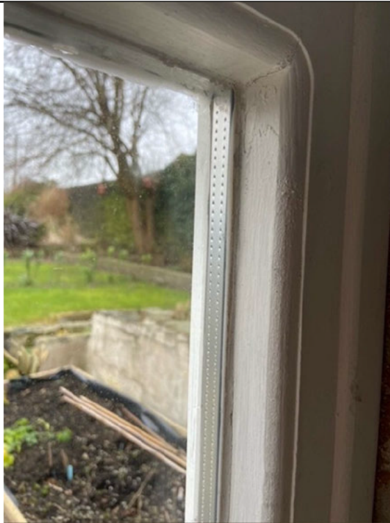
Internal lounge window showing existing double glazing
