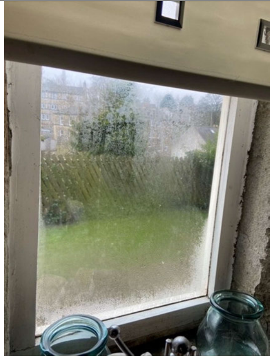
Right hand side internal showing single glazed
