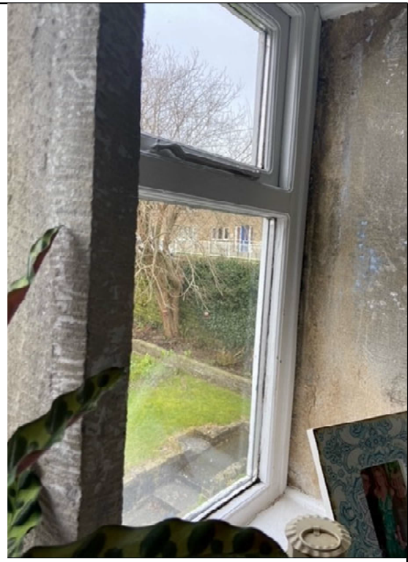
Bedroom 2 showing double glazing
