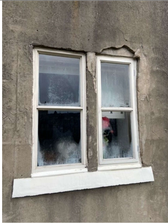
Both windows (external)
