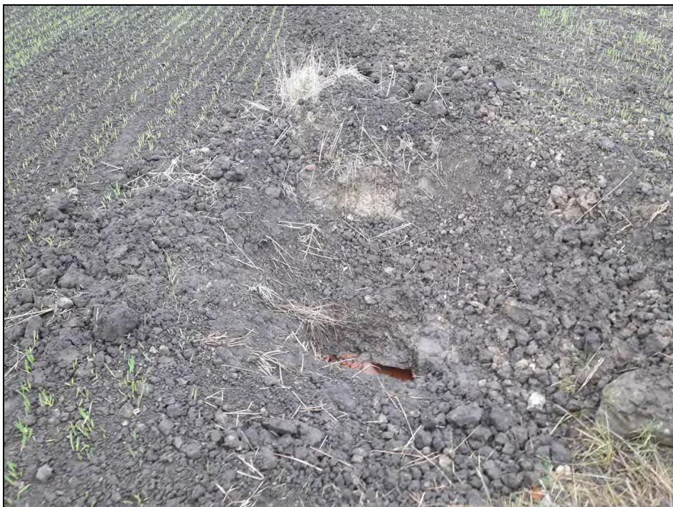
Figure 4 Broken Land Drain
