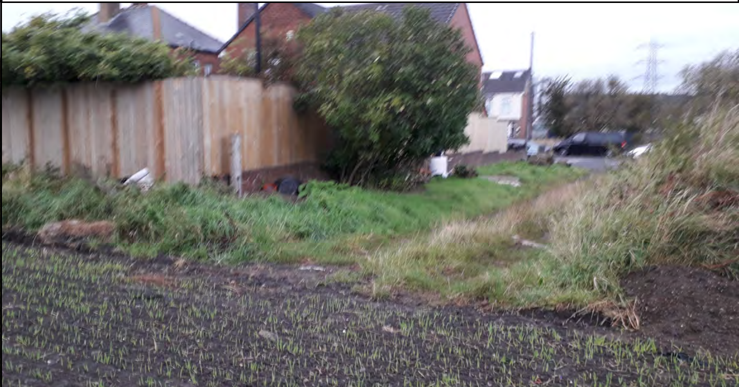
Looking north towards site entrance
