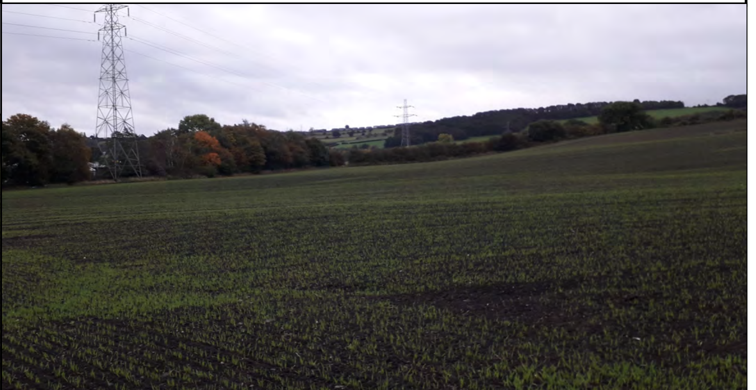
Electricity pylon on eastern boundary
