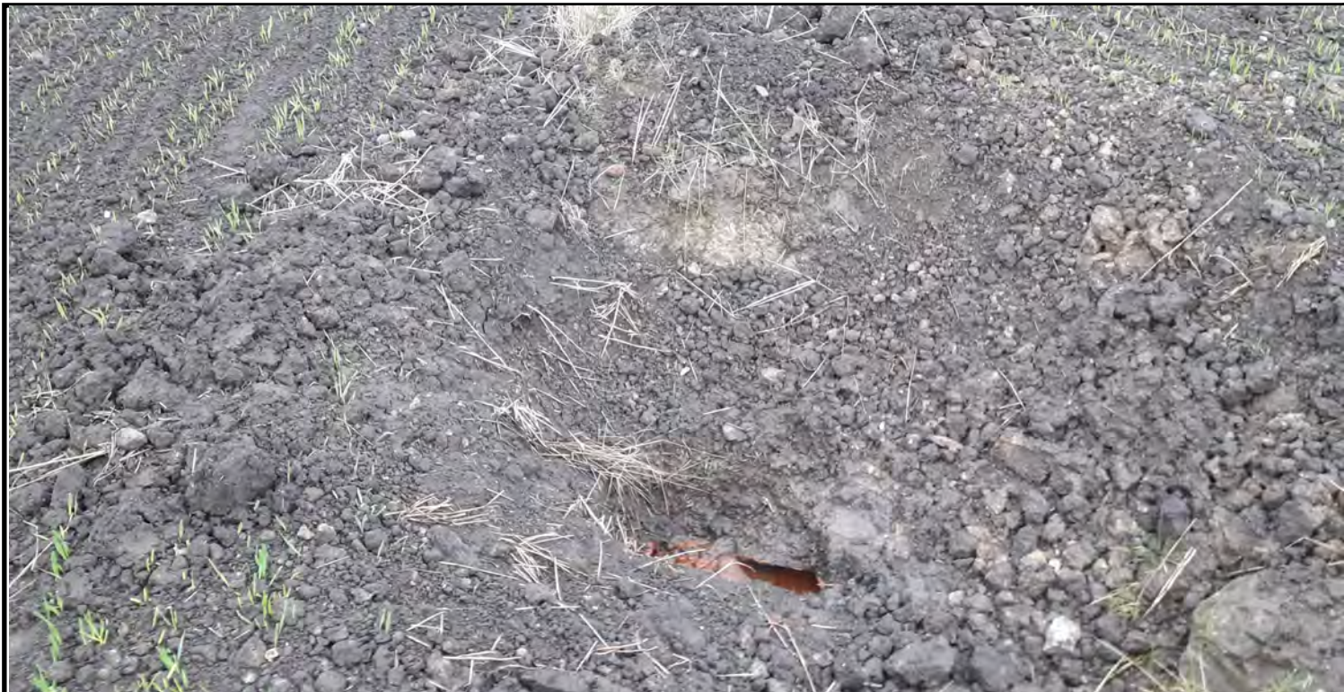
Pit near centre of site with drainage pipe at base
