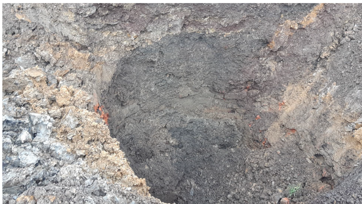
Photo 1: Mine shaft 423419-006. Shaft level approximately 1.45m bgl.
