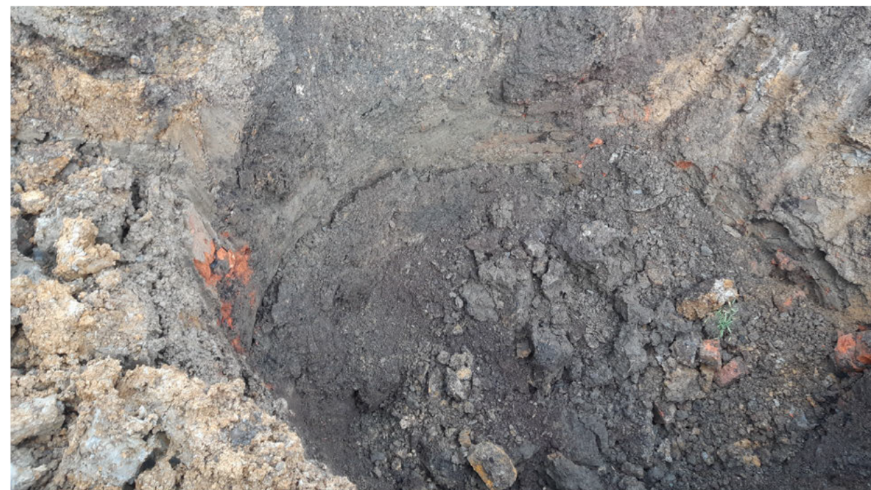
Photo 4: Mine shaft 423419-006. Shaft infilled with soil. Poor condition. No capping or evidence of treatment.
