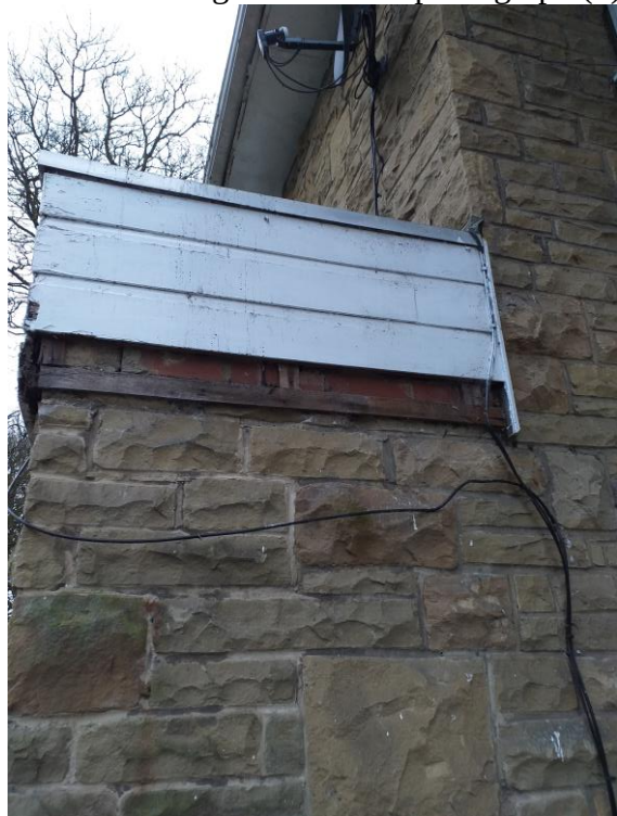
Plastic cladding over brick – photograph (b)
