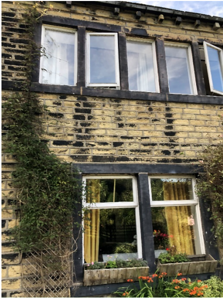
Existing windows and hammer dressed stone.
