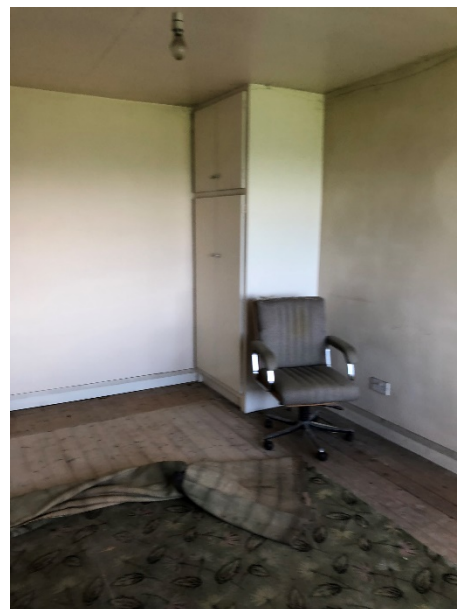
Existing internal ceiling, walls & floor.
