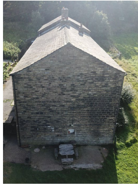
Existing stone roof tiles.
