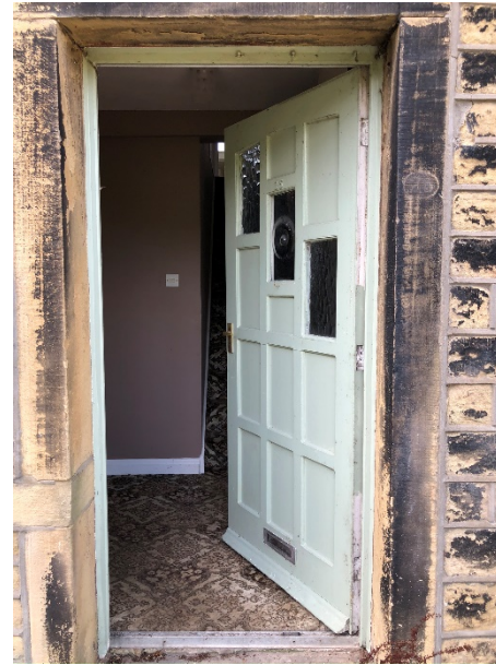
Existing external door.
