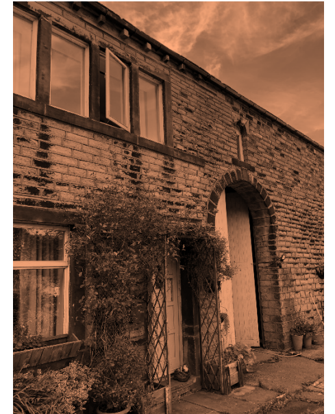
Terrace and attached barn
