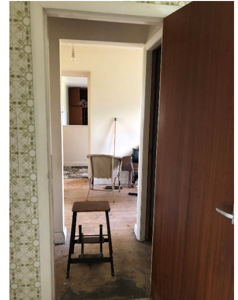
Existing internal door.
