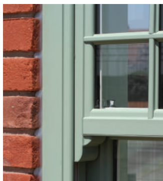
Run through sash horns
