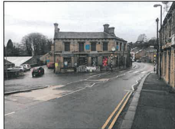
Co-op Convenience Store and Car Park
