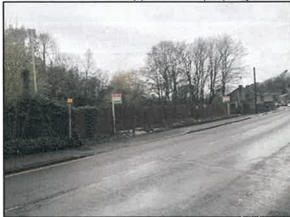
Former Petrol Filling Station Site on North Road – Now vacant
