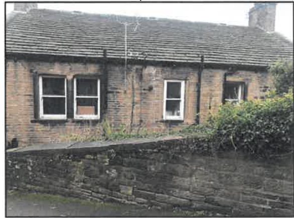
Rear Elevation of Building
