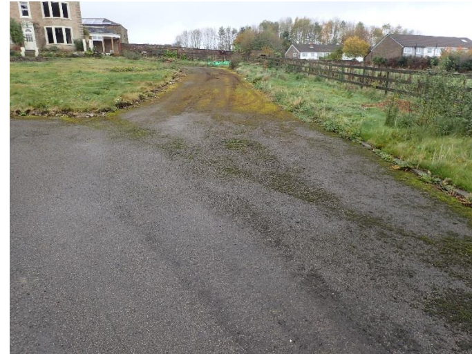
Figure 5 Tarmac driveway leading up to main house
