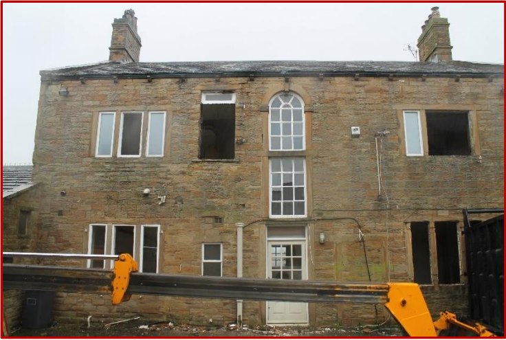
Rear elevation. Rough stone. Central stair lights and showing pitched roof.
