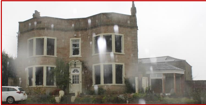
Front elevation. Double bay flat roof projection. Single storey side extension. Use of ashlar stone and quoins.
