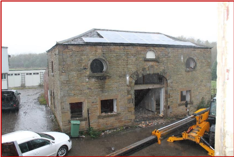
Main barn to rear. Modern buildings are shown to the rear.
