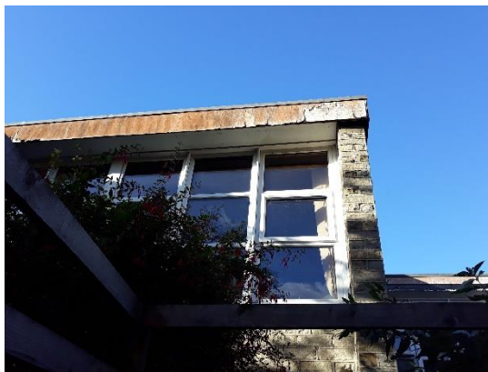
Figure 15_ external window panel to receive new doors
