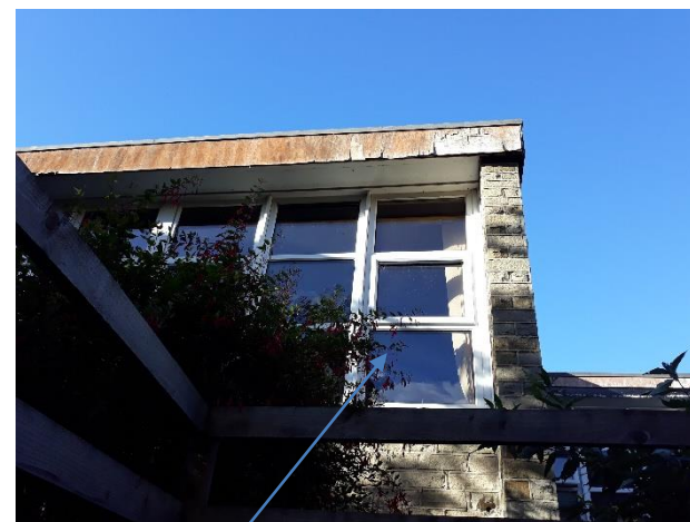
Fig 7: Existing windows to be removed in lieu of new external doors to proposed outside covered space
