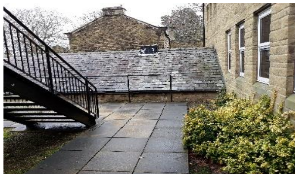
Fig 9: Area being excavated to rear of former Stable Block for proposed steps
