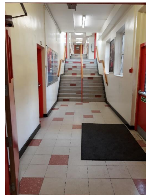
Fig 5: Existing Corridor & steps
