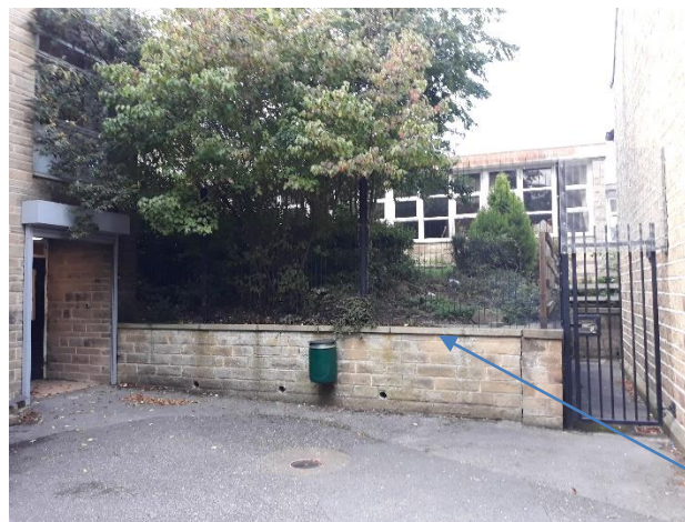
Fig 8: Existing outdoor space adjacent to classroom being remodelled to form additional dining hall space.
