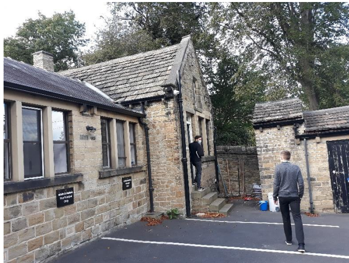
Fig 20: Former Stable Block – front elevation is a later addition with fenestration and stone infill
