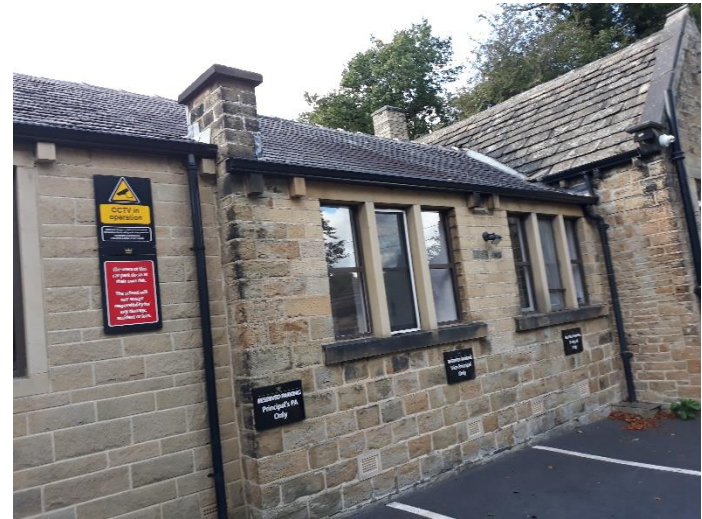
Fig 21: Modern stone infill (to left hand side) earlier parts of building to right hand side now occupied as caretakers office
