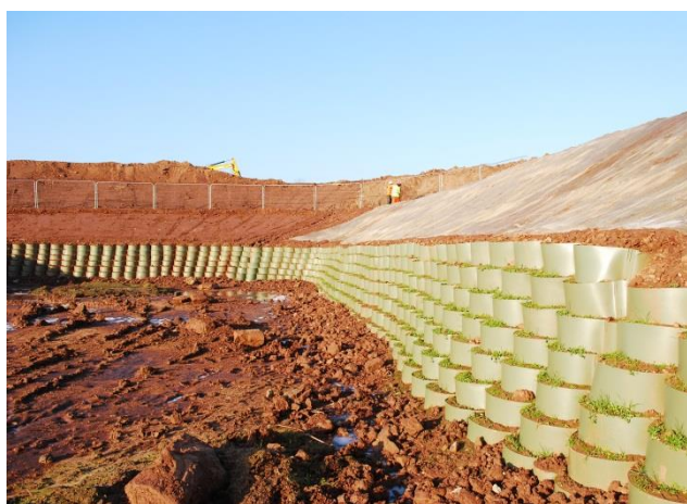
Finished structure with upper slopes reinforced with Abgrid and surface protected with Erosamat Type 1
