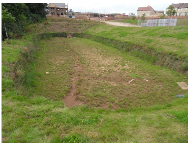
Finished pond starting to green and blend with the natural environment
