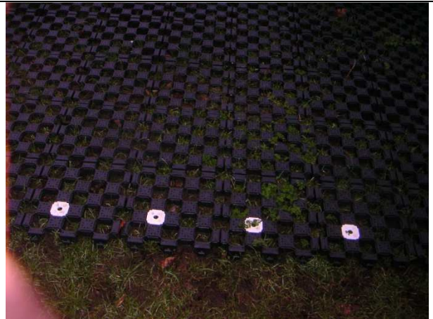
Photo 8: mesh grid laid down for temporary car park.
