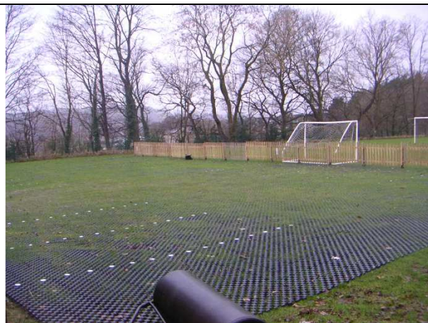
Photo 5: View of width of temporary car park.
