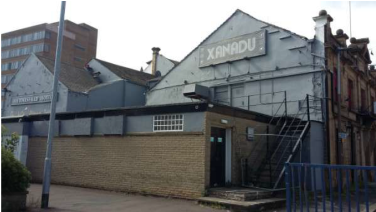
View of part buildings from Southgate ring road
