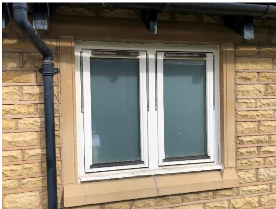
Photo 18 – Replacement windows elsewhere on site
