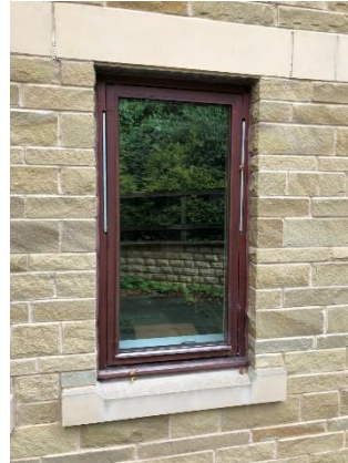
Photo 17 – Replacement windows elsewhere on site
