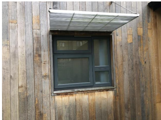
Photo 19 – Replacement windows elsewhere on site
