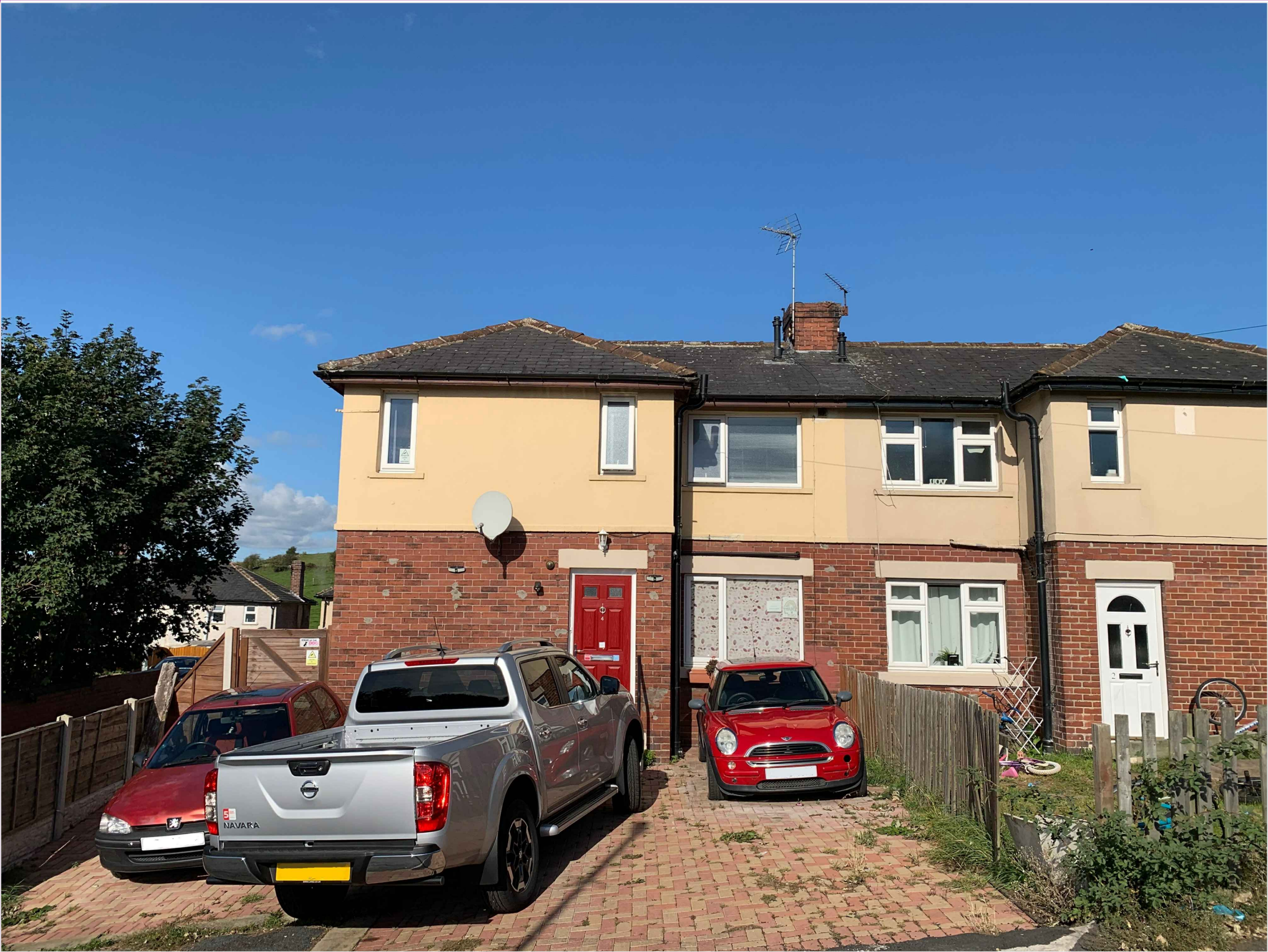
View of south-east facing elevation (front of property)
