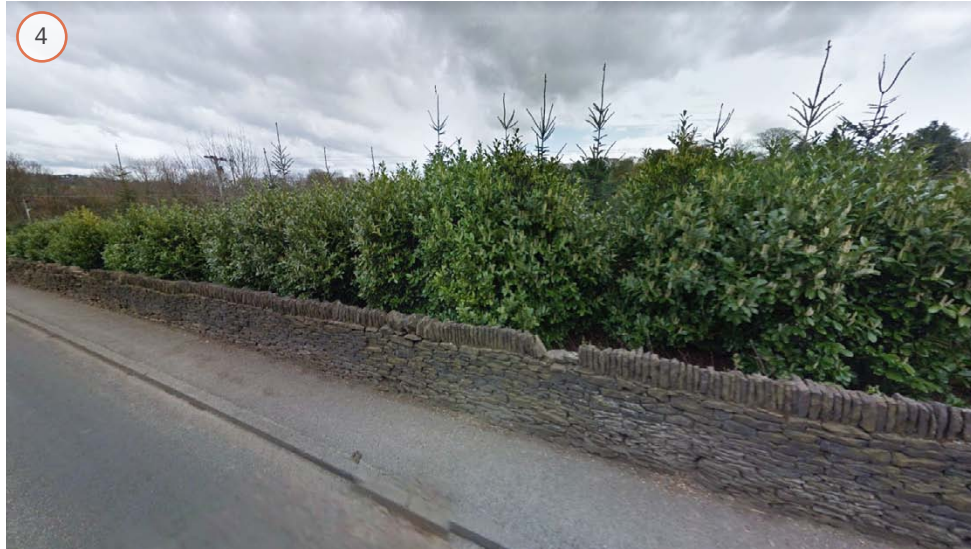
EXISTING VEGETATION & WALL FACING ABBEY ROAD ON THE WEST BOUNDARY OF THE SITE.
