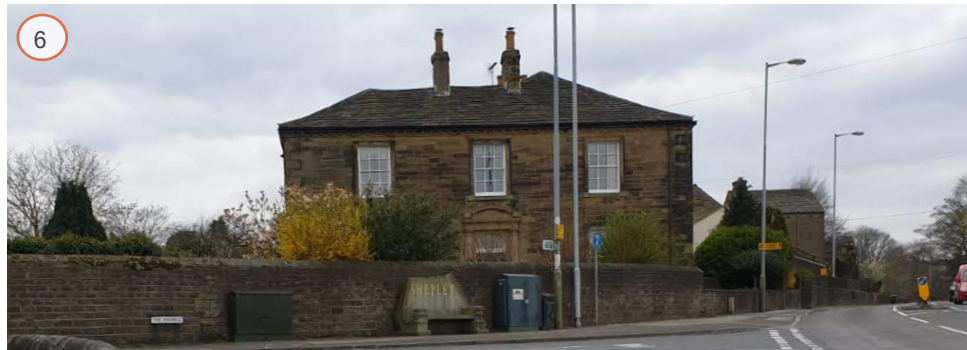
END OF TERRACE, STONE PROPERTY AT THE JUNCTION OF ABBEY ROAD & THE KNOWLE
