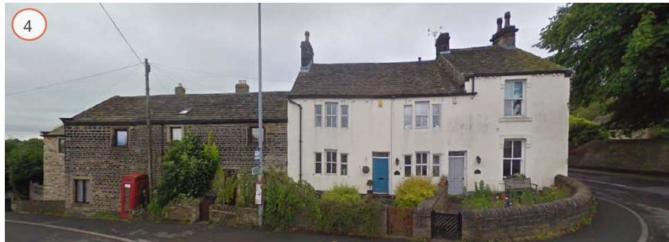
FRONT OF STONE AND RENDER TERRACES SOUTH OF THE SITE
