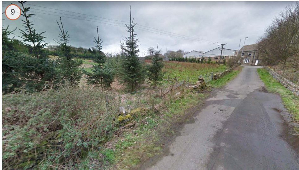
DILAPIDATED BOUNDARY TREATMENT ALONG THE KNOWLE
