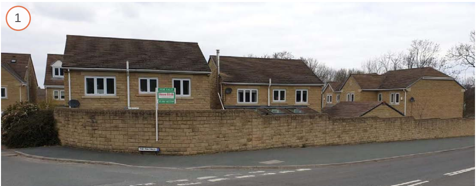
DETACHED, STONE PROPERTIES DIRECTLY OPPOSITE SITE, BACKING ON TO ABBEY ROAD
