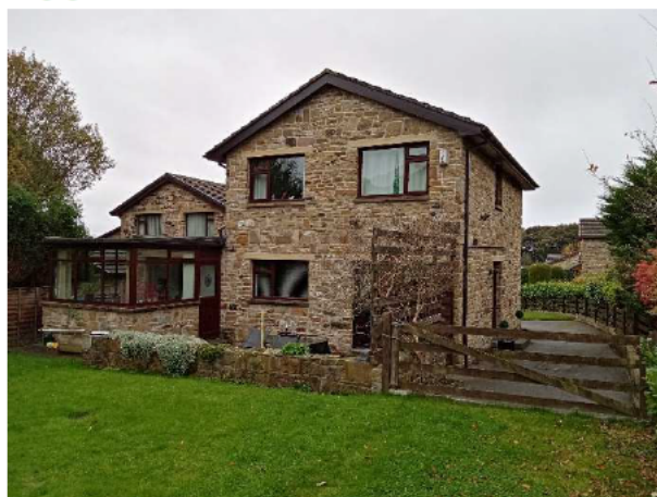
Photo 2: Rear of the house viewed from the north.
