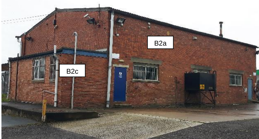
Photograph 9: North eastern aspect of B2.
