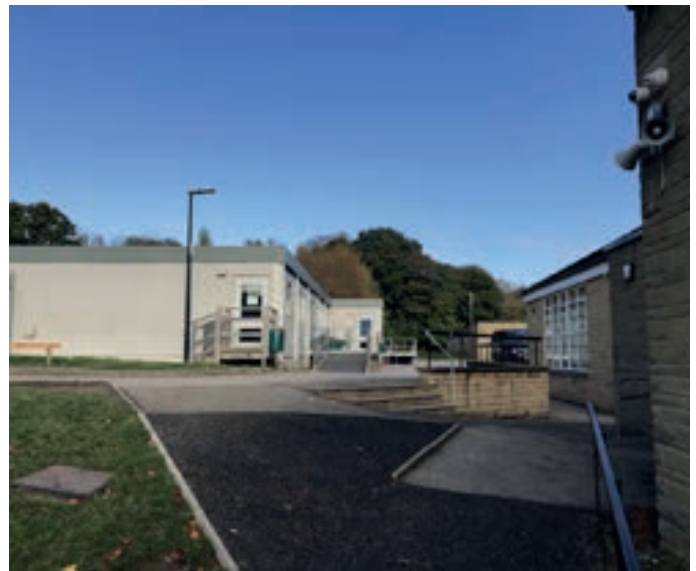
4: View from the sports hall facing the temporary units, showing the external level change.
