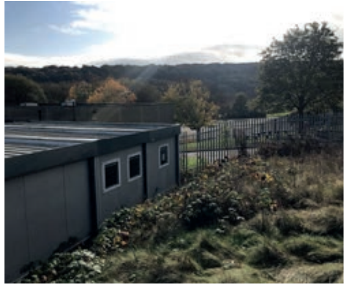
7: Rear view from the back of the site towards rear access of the temporary units.
