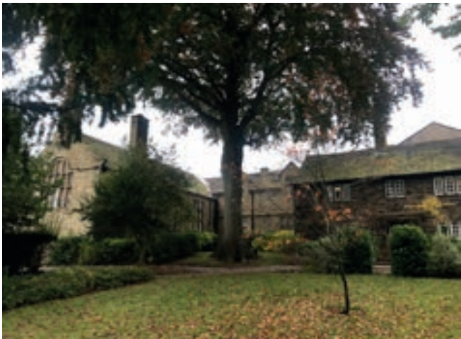
PHOTO 18: View from the front elevation
