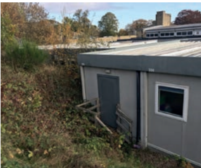
10: View from the rear of the site showing the back of the temporary classroom proposed for removal.
