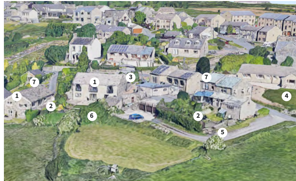
EXISTING EXAMPLE: GOLCAR, HUDDERSFIELD
