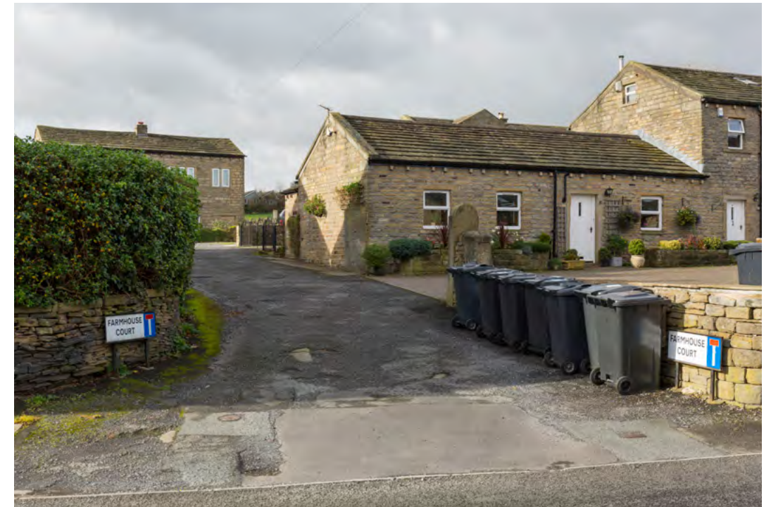
10. GLIMPSED VIEW THROUGH LISTED BUILDINGS AT FARMHOUSE COURT
