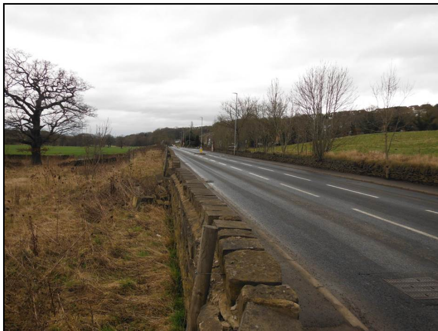
Photograph 9: View N along Penistone Road from location E.
