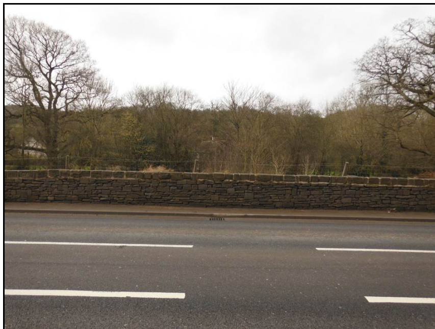
Photograph 11: View towards the LB from location F.
