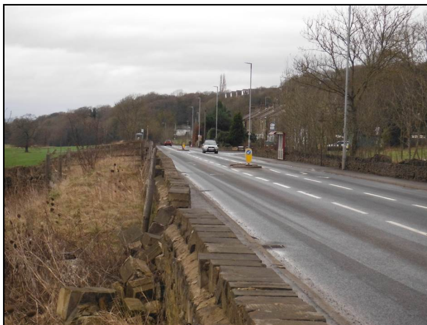
Photograph 10: Zoomed view as above towards the proposed new roundabout location.
