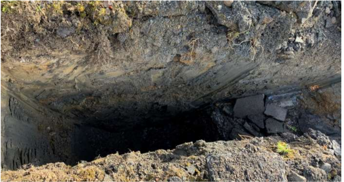
Photo 1: TP1 at a maximum depth of 3.00mbgl.
