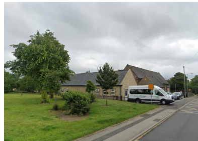
Primary School extensions
