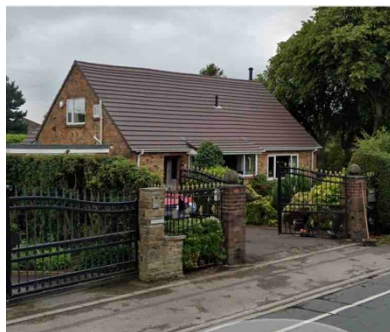
Brickwork of bungalow adjacent to Memorial
