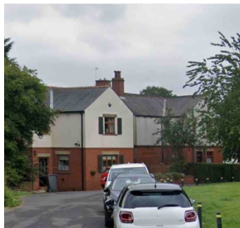
Brickwork of houses adjacent to site
