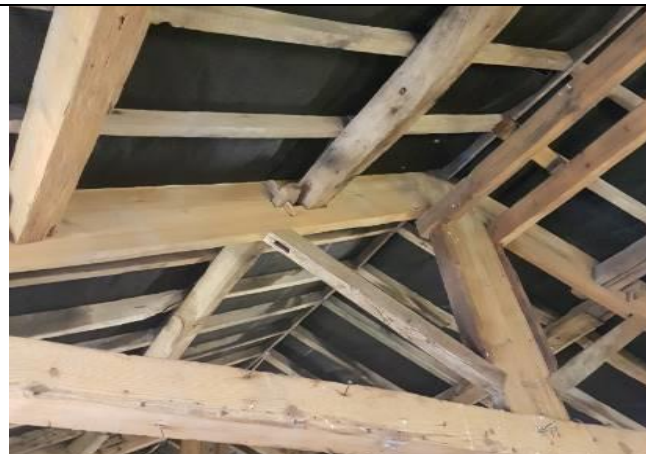
Photo 5: Recently installed roof liner in building 1.
