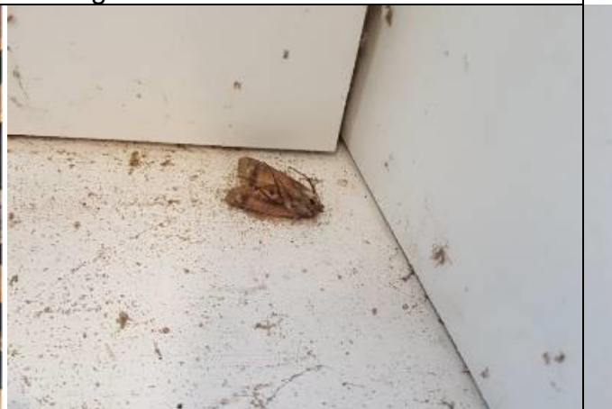
Photo 6: Intact moth within building 1.
