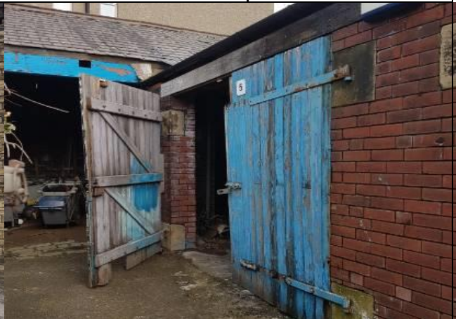
Photo 24: Access into building 4.
