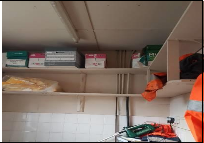
Photo 20: Fake roof installed within building 5.
