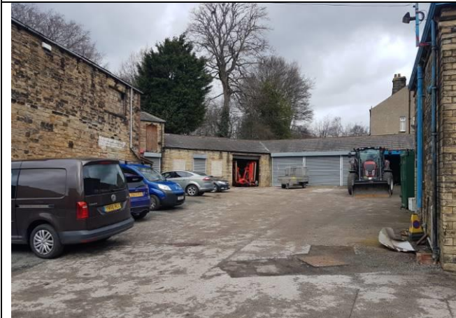
Photo 23: Hard standing carpark council vehicle storage.
