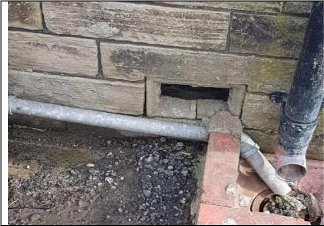
Photo 19: Airbrick towards ground level of building 5.
