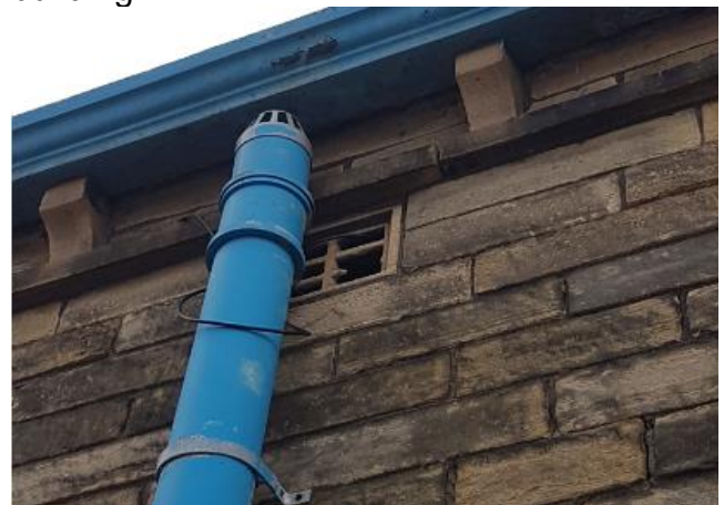
Photo 18: Airbrick towards roof of building 5.
