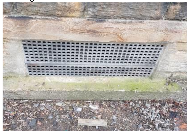
Photo 3: Airbrick at ground level of building 1.
