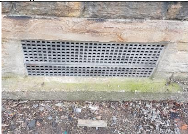
Photo 3: Airbrick at ground level of building 1.
