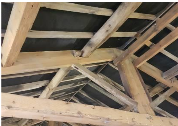
Photo 5: Recently installed roof liner in building 1.
