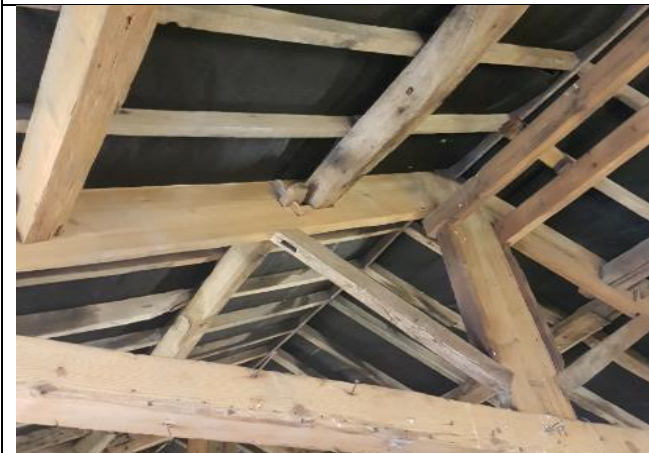
Photo 5: Recently installed roof liner in building 1.
