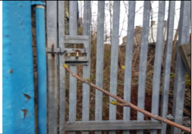
Photo 22: Scattered scrub with no access available for detailed inspection.
