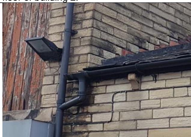
Photo 12: Lifted roof tiles at eaves of building 3.
