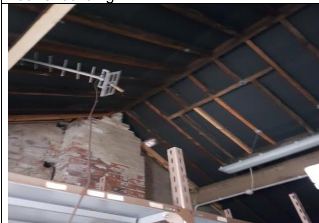
Photo 9: Timber framed roof with roof liner in building 2.
