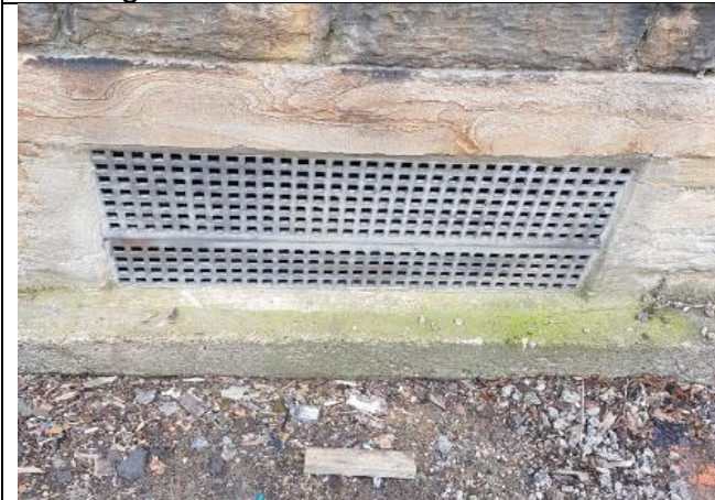
Photo 3: Airbrick at ground level of building 1.
