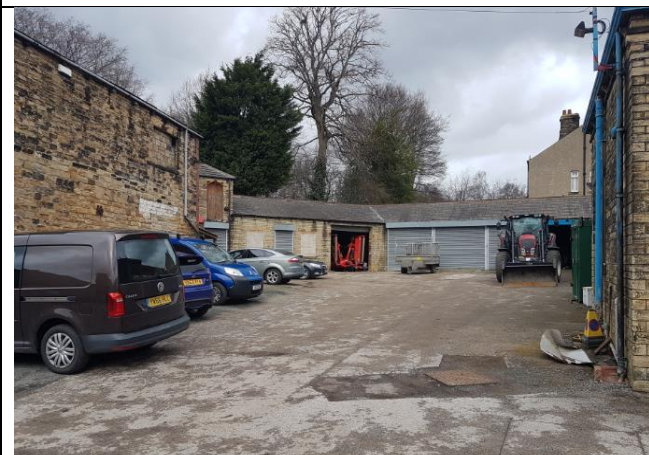
Photo 23: Hard standing carpark council vehicle storage.
