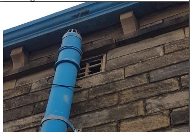
Photo 18: Airbrick towards roof of building 5.
