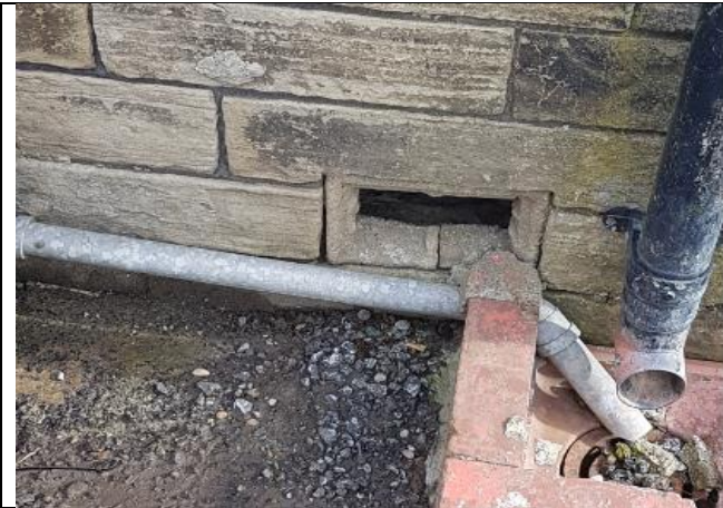
Photo 19: Airbrick towards ground level of building 5.
