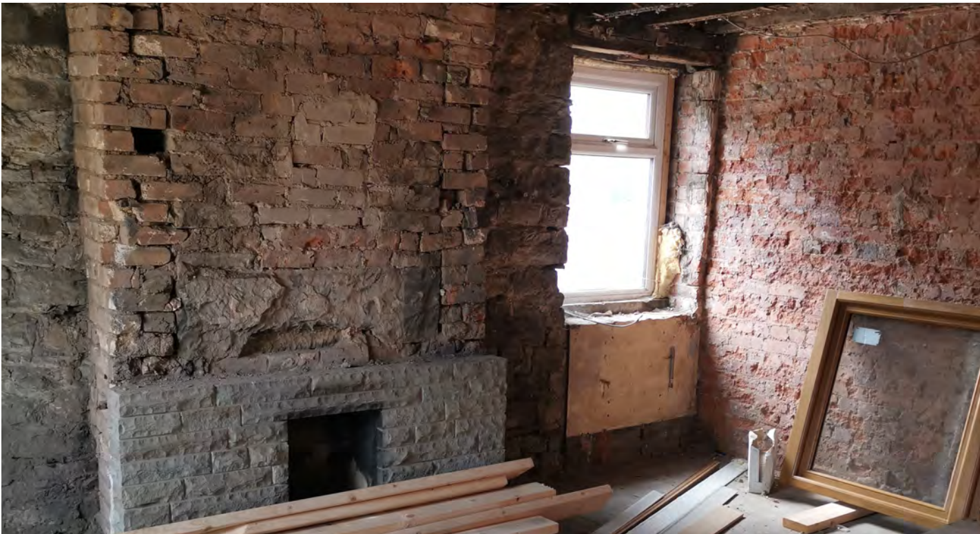
IMAGE 7_ IMAGE ILLUSTRATING REBUILDING OF NORTH FAÇADE IN RED BRICK.
