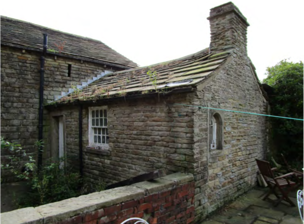
IMAGE 4_ VIEW OF FORMER SINGLE STOREY BUILDING ATTACHED FORMING PART OF THE ASSET’S LISTING. DEMOLISHED DURING THE DEVELOPMENT OF PARK FARM.
