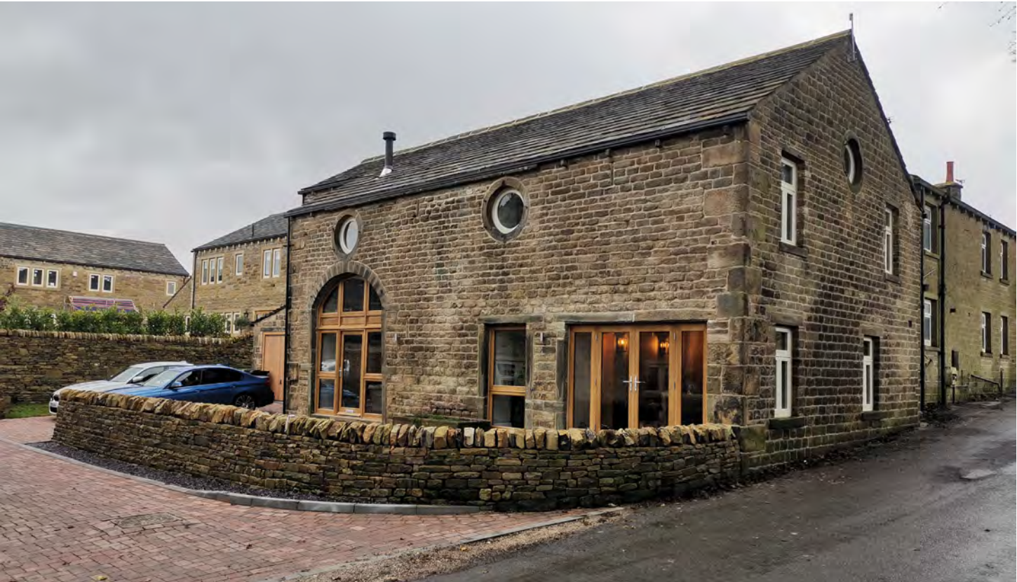
IMAGE 19_ VIEW FROM ENTRY TO PARK FARM MEWS WHERE THE ASSET’S HISTORY, SIGNIFICANCE AND ARCHITECTURAL MERIT CAN BE MOST EXPERIENCED AND ENJOYED.
