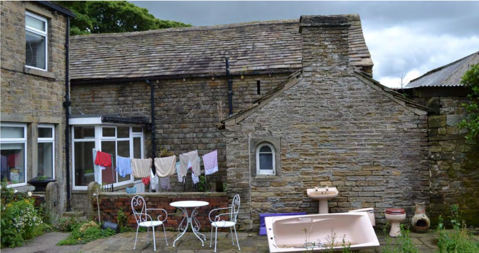
IMAGE 17_ FORMER SINGLE STOREY BUILDING ATTACHED TO THE LISTED BARN, PRIOR TO BEING DEMOLISHED.
