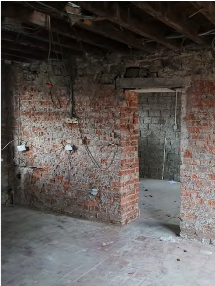
IMAGE 10_ PARTIAL REBUILD OF EAST GABLE IN RED BRICK.
