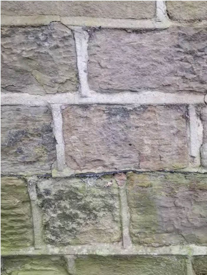
IMAGE 8_ MODERN DPC TO NORTH FACADE
