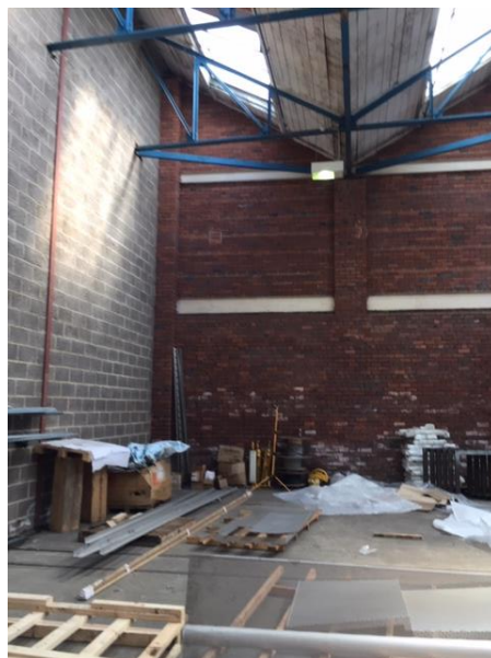
Plate 8-Wall close to blockwork partition
