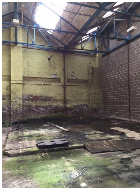
Plate 11- Wall continues to rear of blockwork separating wall
