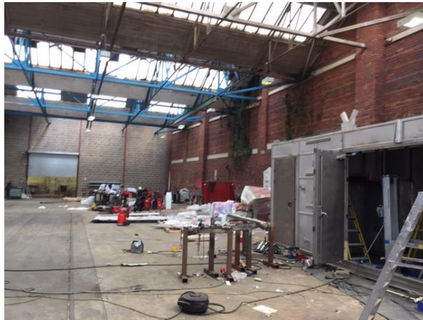
Plate 6-Internal wall looking to the back.
