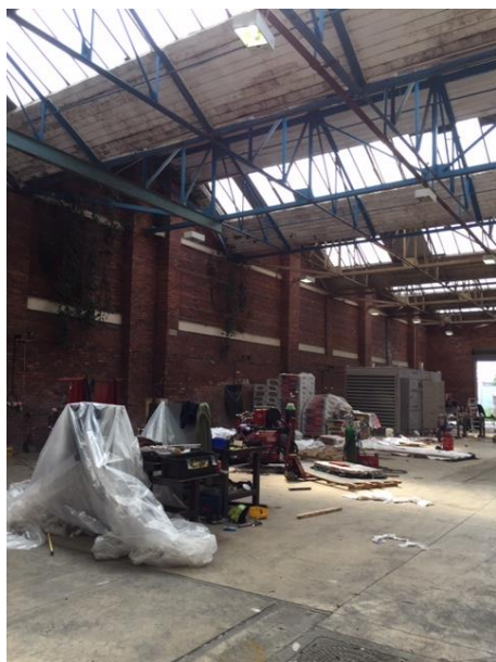
Plate 7-Internal wall looking to the front.
