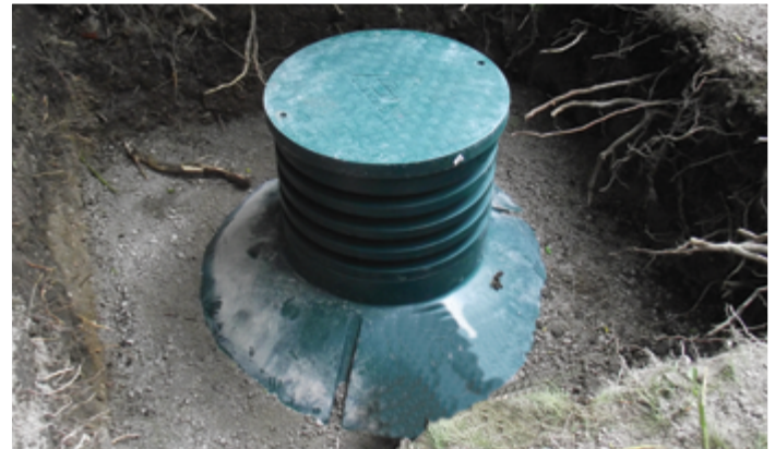
Turret invert extension during installation
