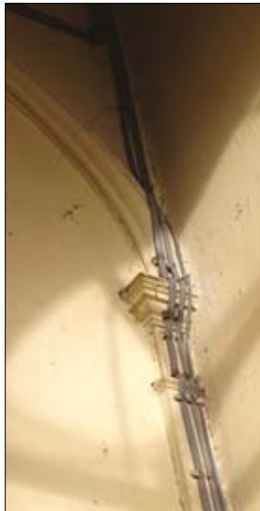
Fig. 15. The mouldings on the original arched entrance to the chapel from the lobby within the central lobby
