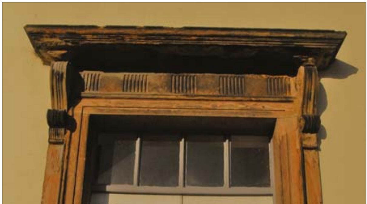
Fig. 16. Moulding on one of the main external entrances
