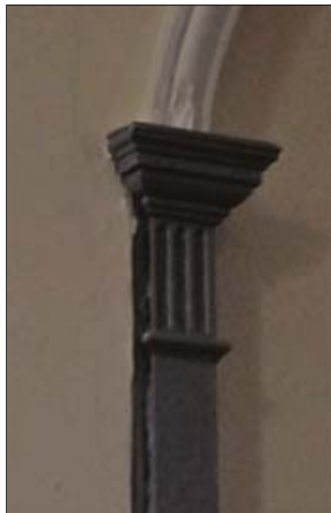
Fig. 14. The mouldings on the original arched entrance to the chapel from the lobby within the chapel
