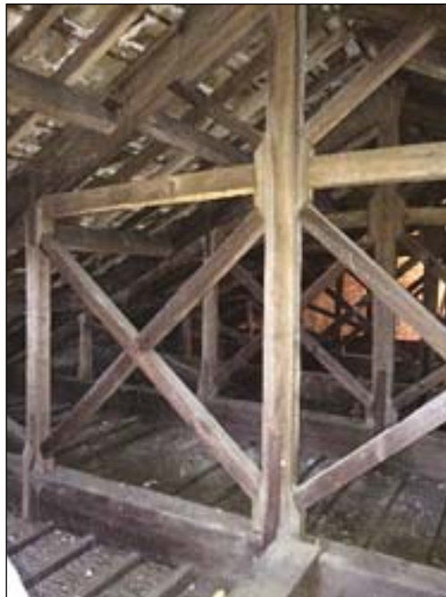
Fig. 12. The interior of the roof space showing the trusses
