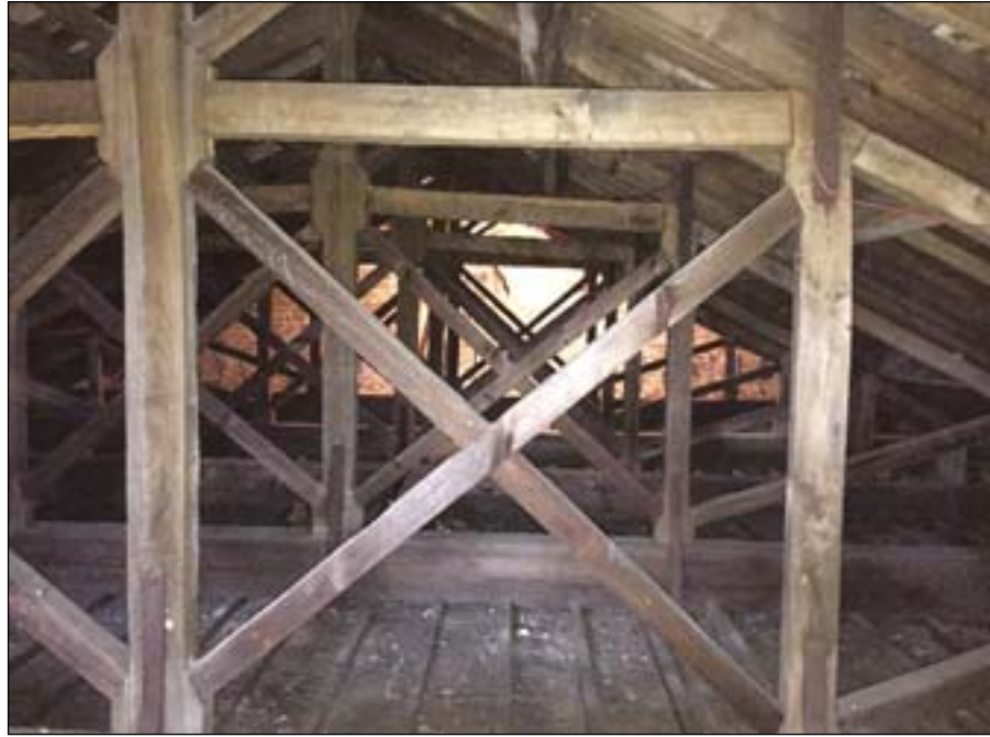
Figs. 11. The interior of the roof space showing the trusses
