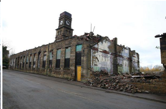
View on Ruth Street towards SW post demolition
