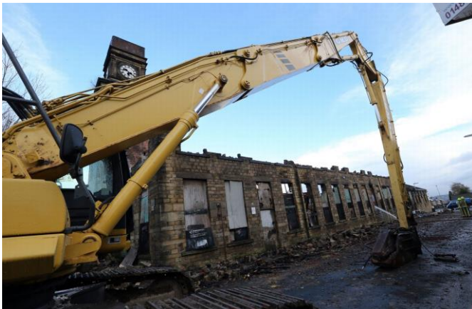
View along Ruth Street towards NE during demolition
