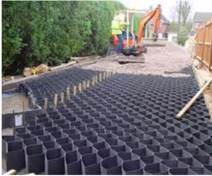
Figure.2. Example Cellular Confinement System (CCS)
