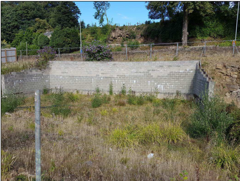
Photograph 8: Looking at the retaining wall and structure at the western boundary of the site.
