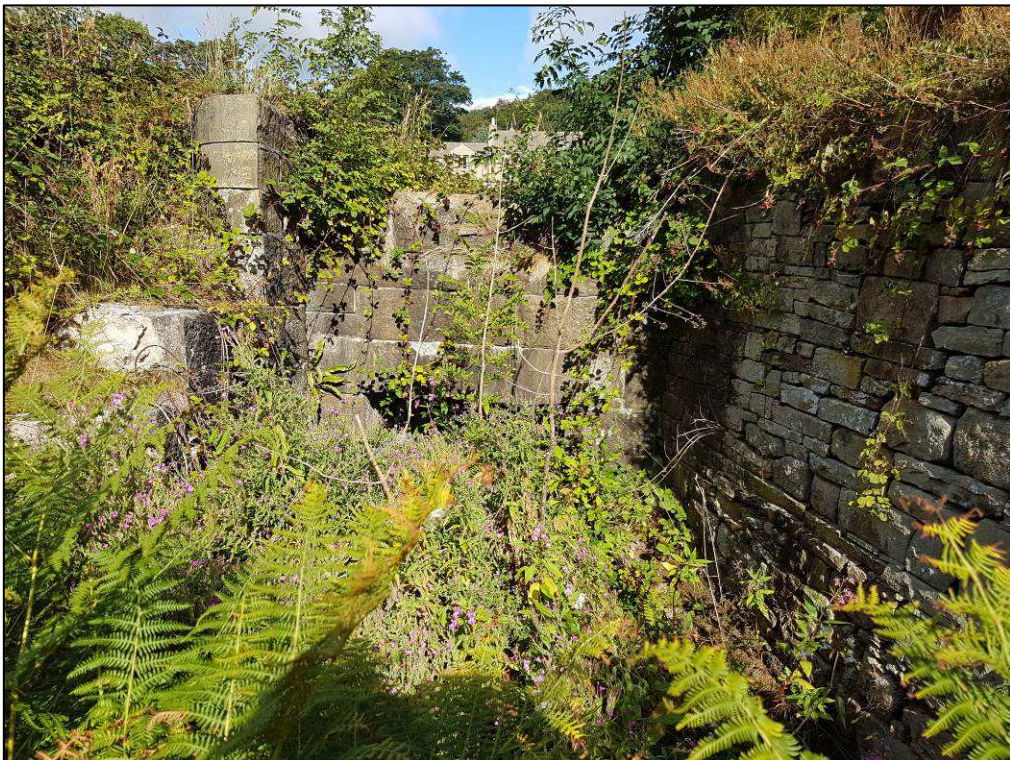
Photograph 12: Looking west at the inactive/historical sluice.
