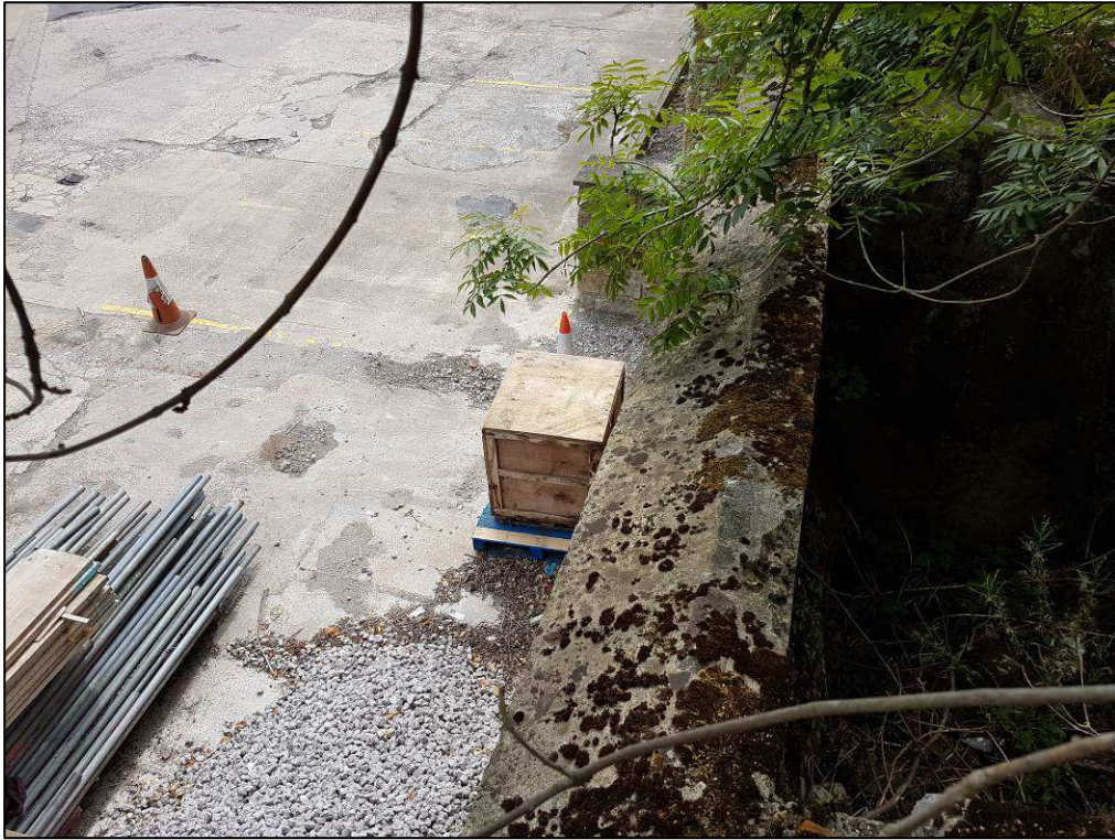
Photograph 11: Looking down from the top of the retaining wall located at the northern end of the site.
