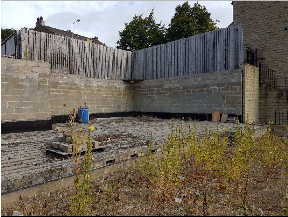
Photograph 7: Looking at the beam and block floor and retaining wall at the western boundary of the site.
