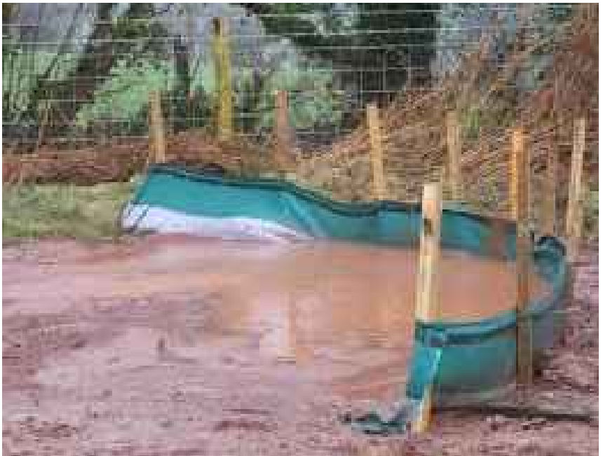
HY-TEX TERRASTOP SILT FENCING TO BE INSTALLED TO MANUFACTURERS SPECIFICATION (refer to manufacturers installation guidance)
