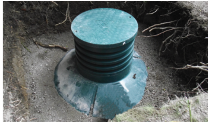
Turret invert extension during installation
