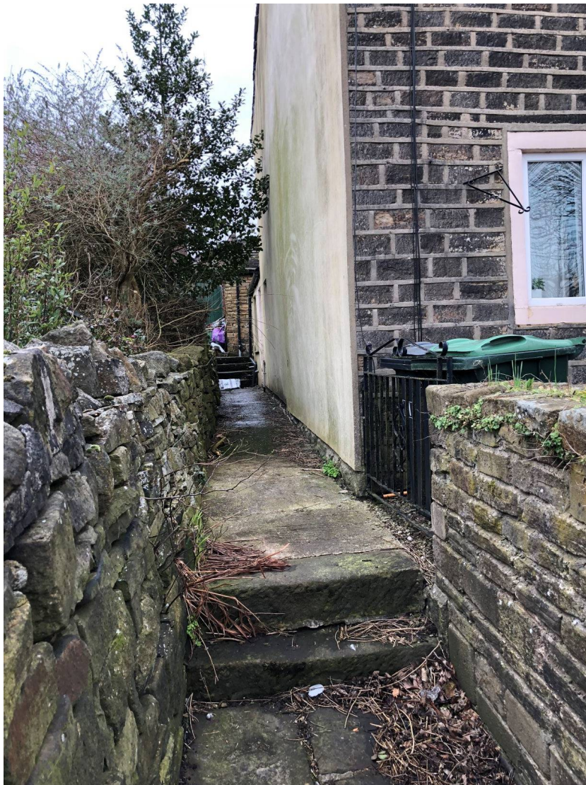
Image 4 - Path to No. 39/41 to be maintained.
