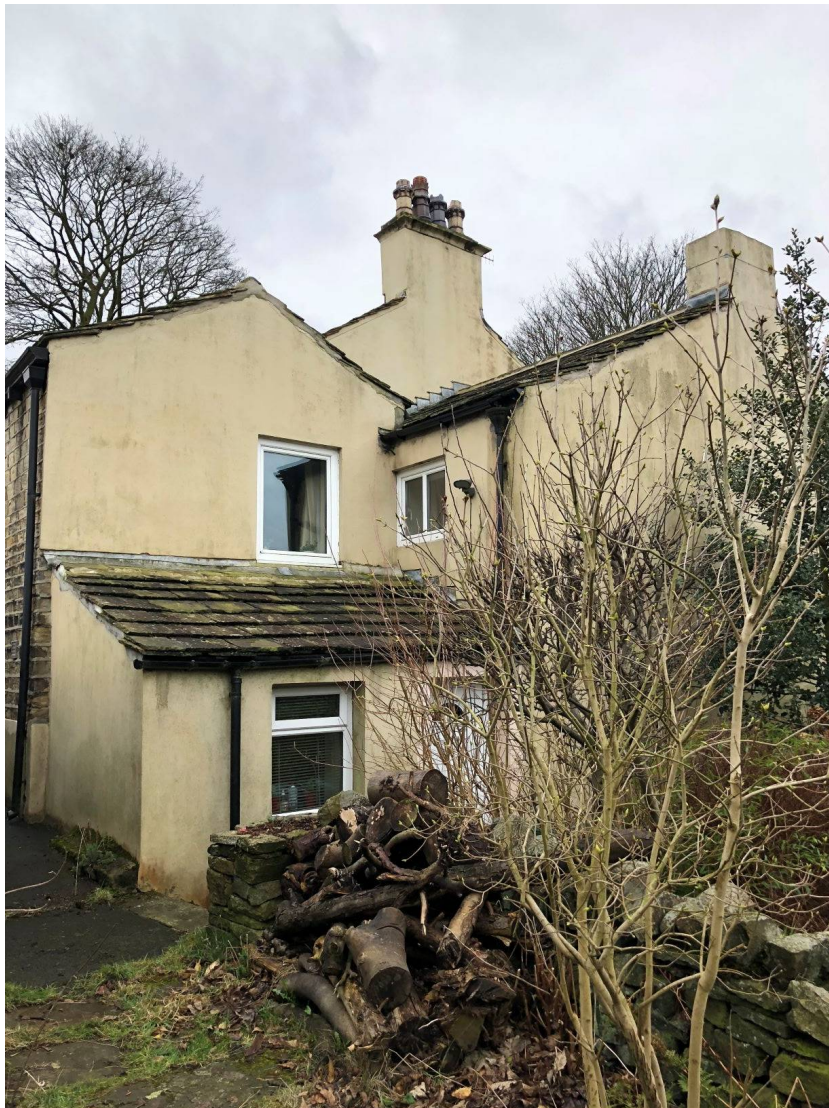
Image 3 - No.39/41 with Habitable Windows to Ground Floor Kitchen and First Floor Bedroom
