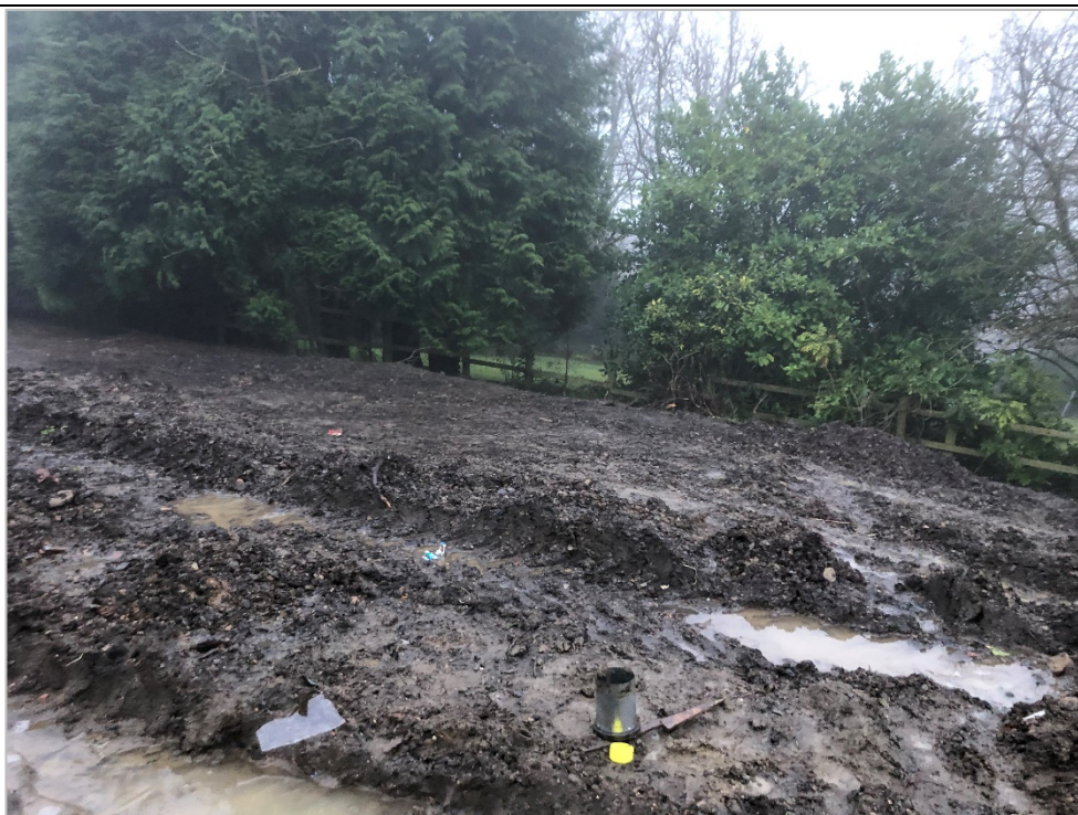
Figure 2 Looking towards the southern part of the site
