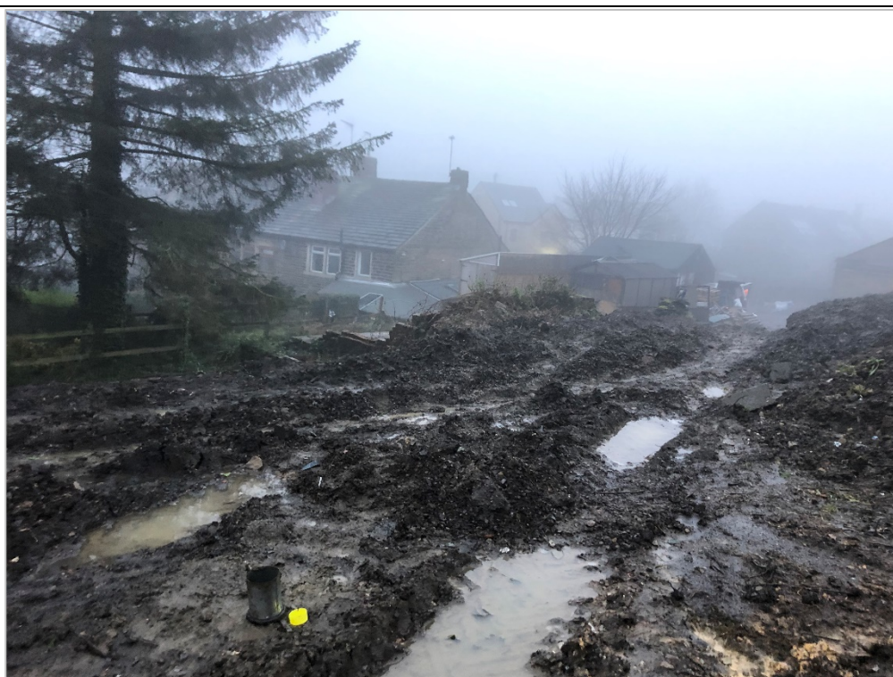
Figure 3 Looking southeast across the site
